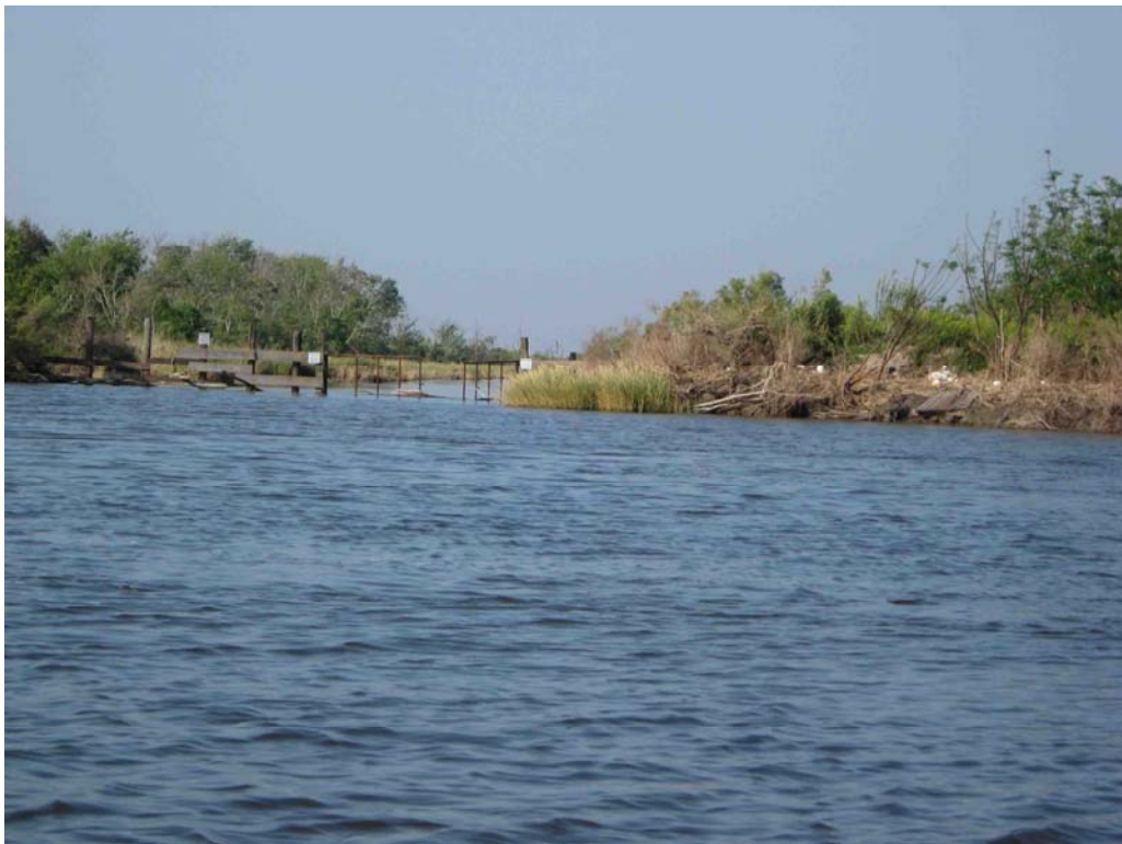
Photo #2 – Access Canal Gate to Water Control Structure.
