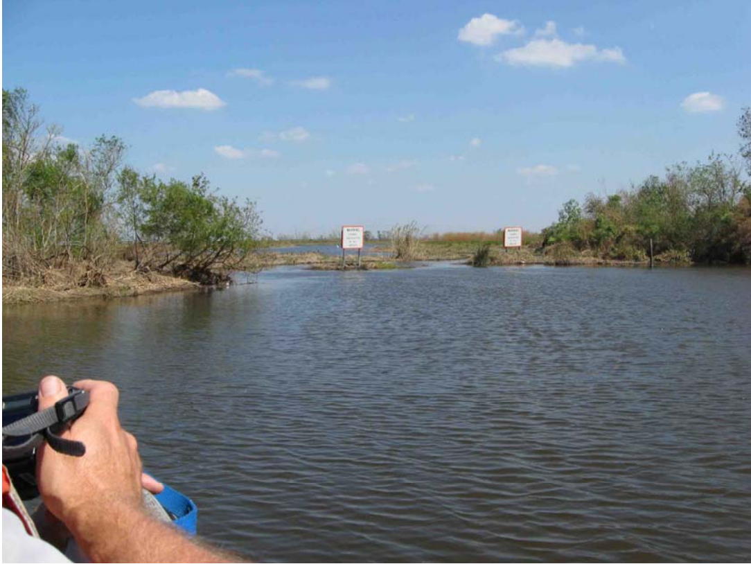
Photo #1 – Structure #14 (Note Gaps)
