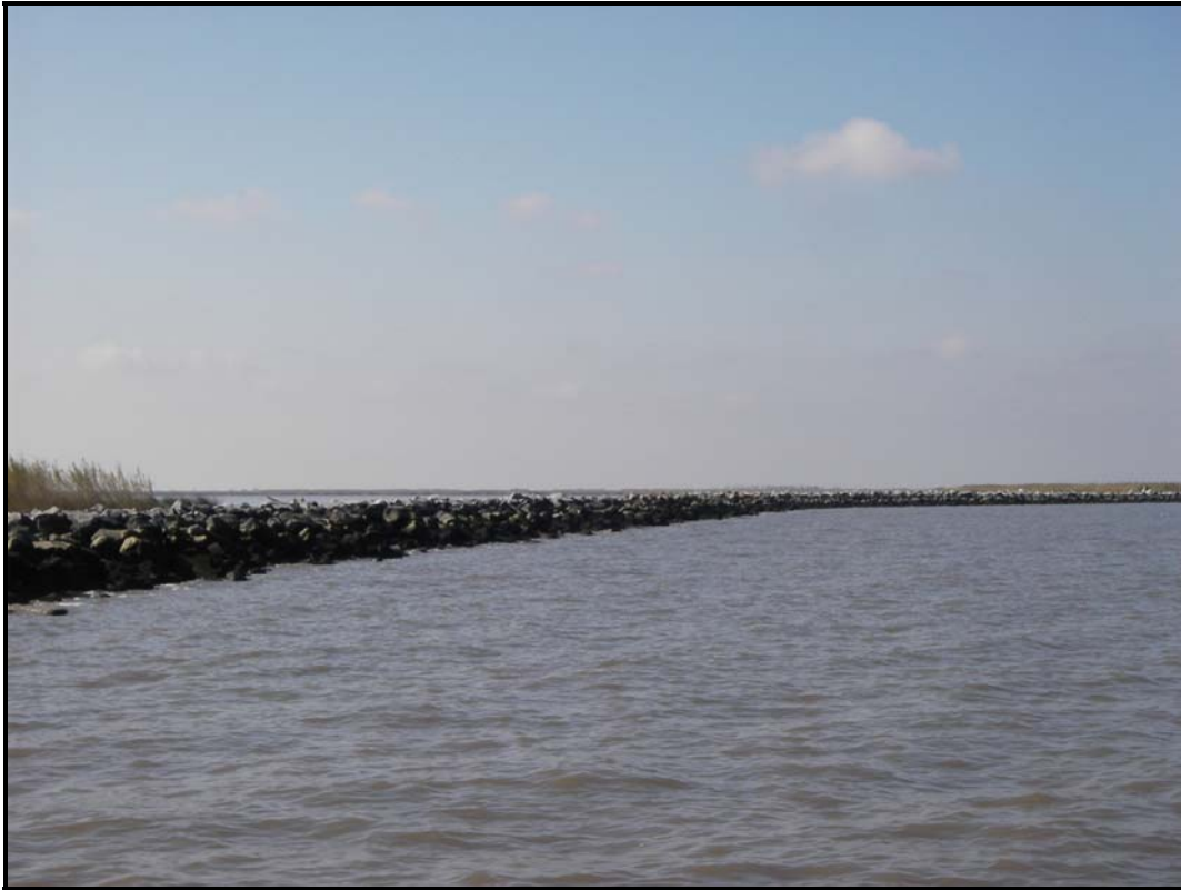
Photo No. 5 , Closure No. 4 looking west
