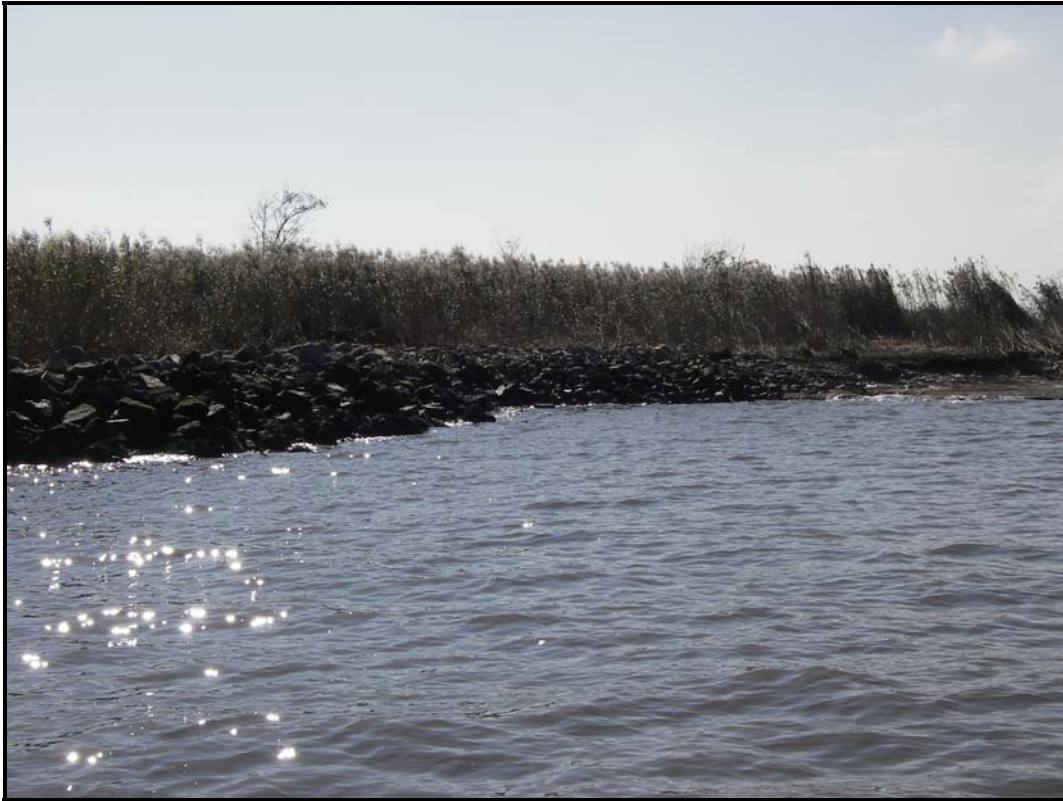
Photo No. 3, Closure No. 3 bank paving west side
