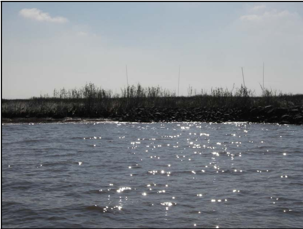
Photo No. 4, Closure No. 4 bank paving east side
