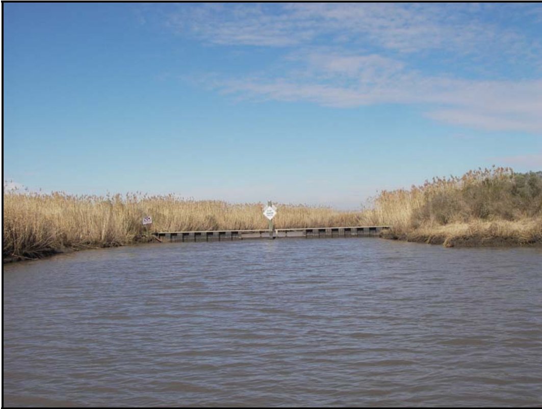
Photo No. 5, Cow Path Structure
