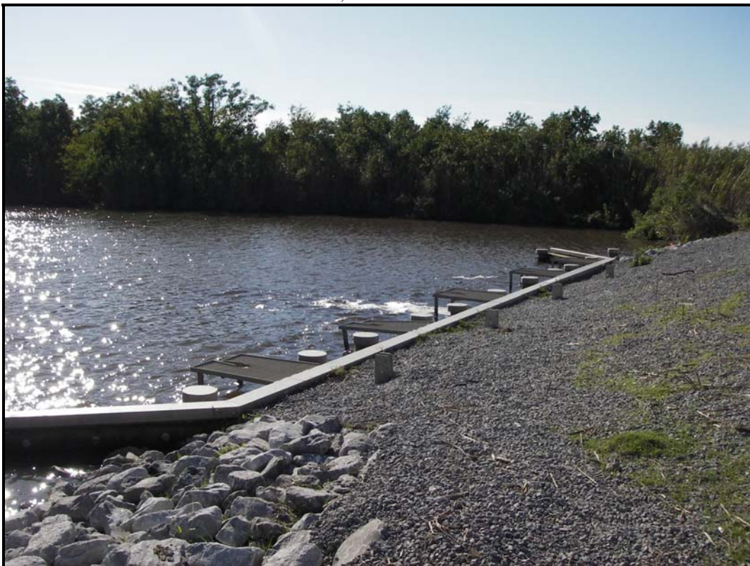
Photo No. 4, Outlet side of structure
