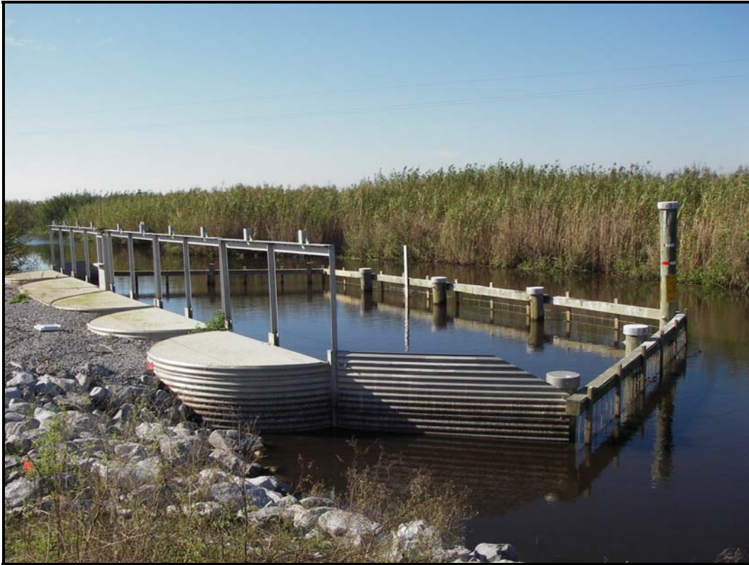
Photo No. 3, Inlet side of structure
