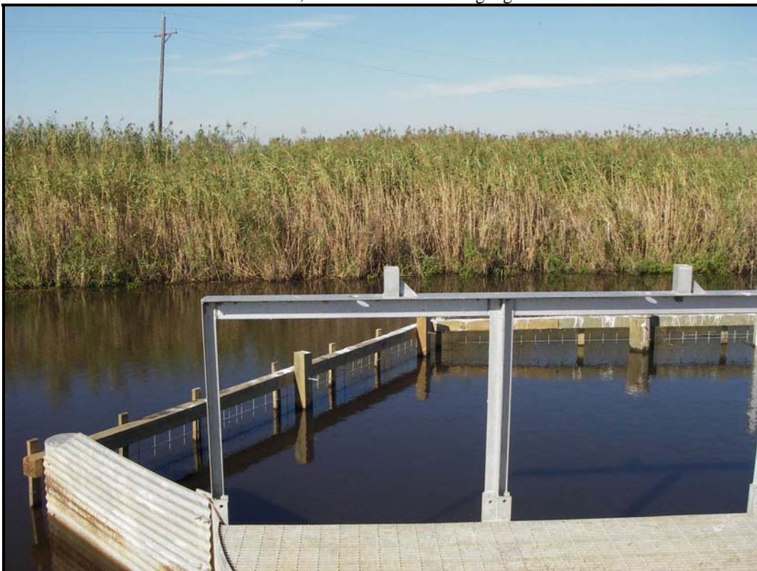
Photo 2, Inlet side showing repairs to hyacinth fence.
