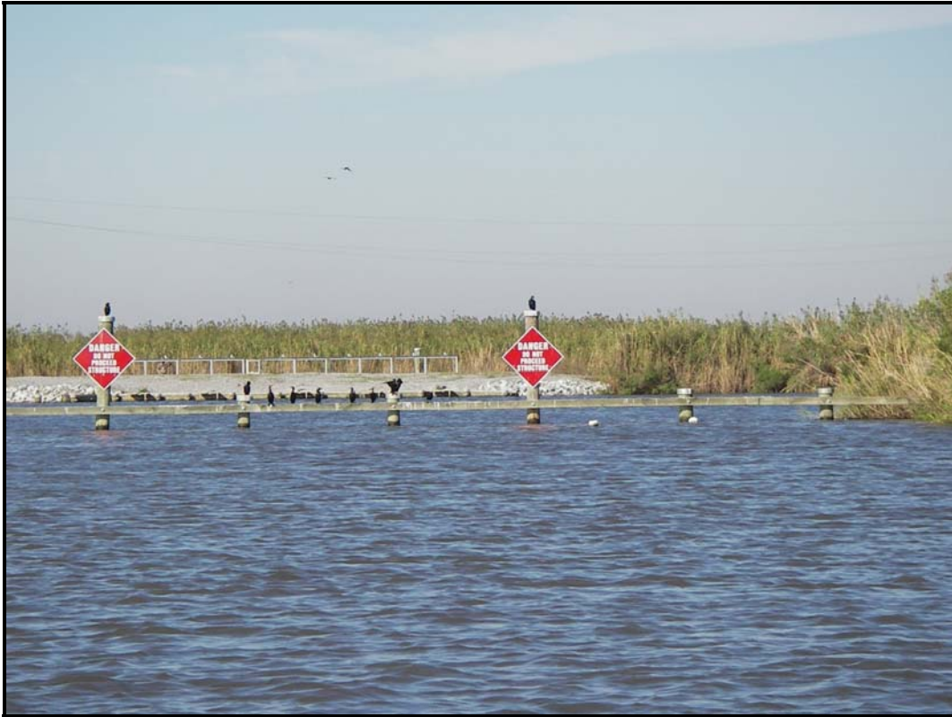
Photo 1, Marine barrier with signage.
