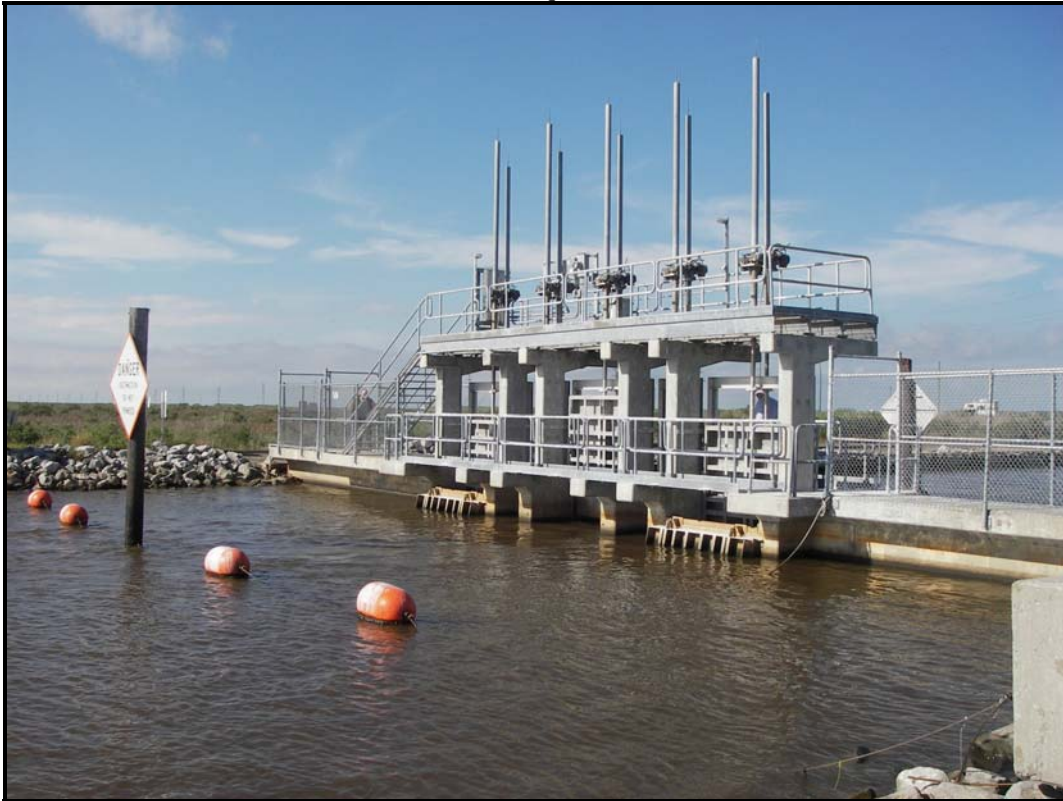
Photo No. 5, West Cove Canal
