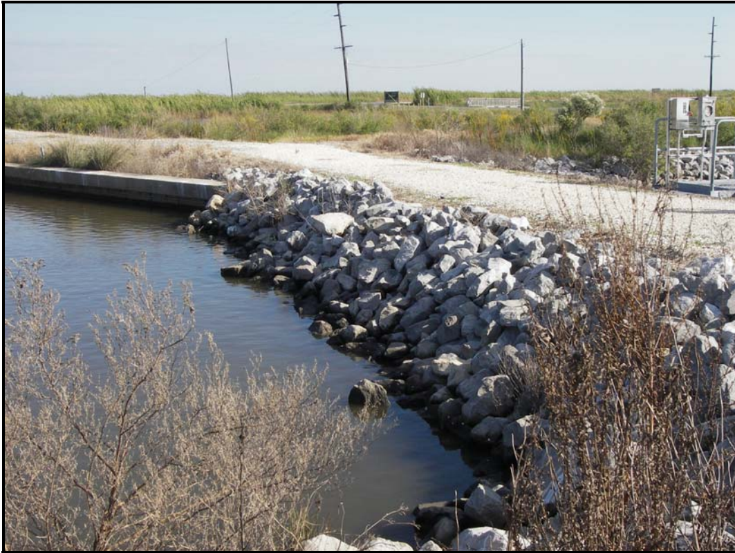
Photo No. 4, Headquarters Structure
