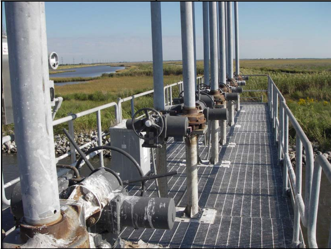
Photo No. 2, Hog Island Gully Structure
