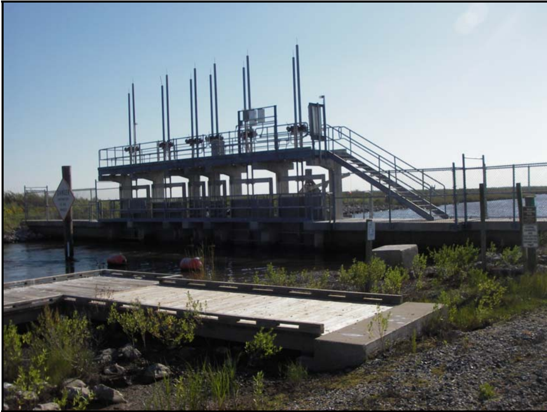
Photo No. 1, Hog Island Gully Structure
