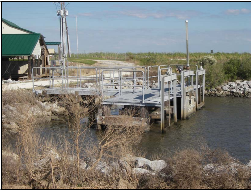
Photo No. 3, Headquarters Structure
