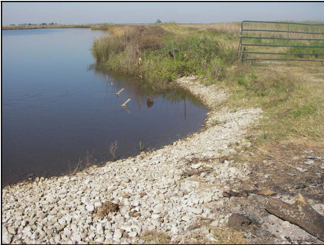
Photo No.3, Structure No.1, outlet side.
