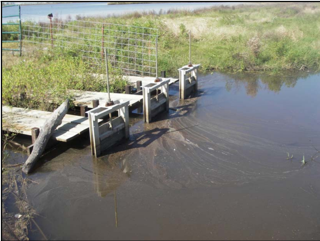
Photo No. 1 , Structure No.1, inlet side.
