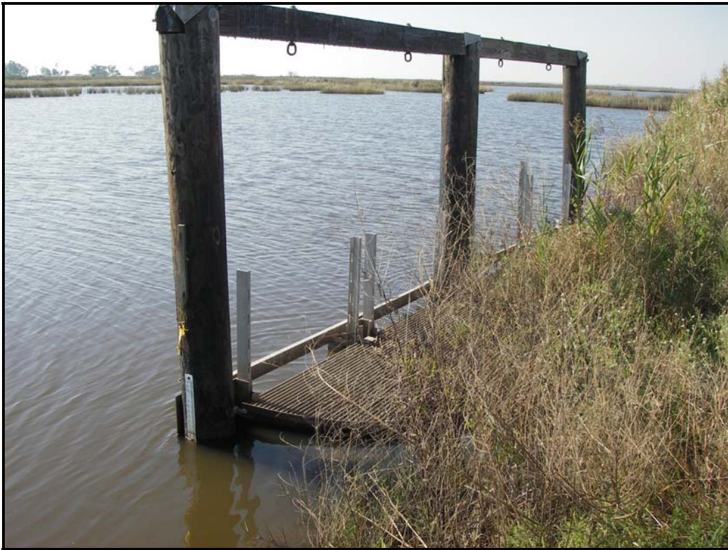
Photo No. 4, Structure No. 12, inlet side.
