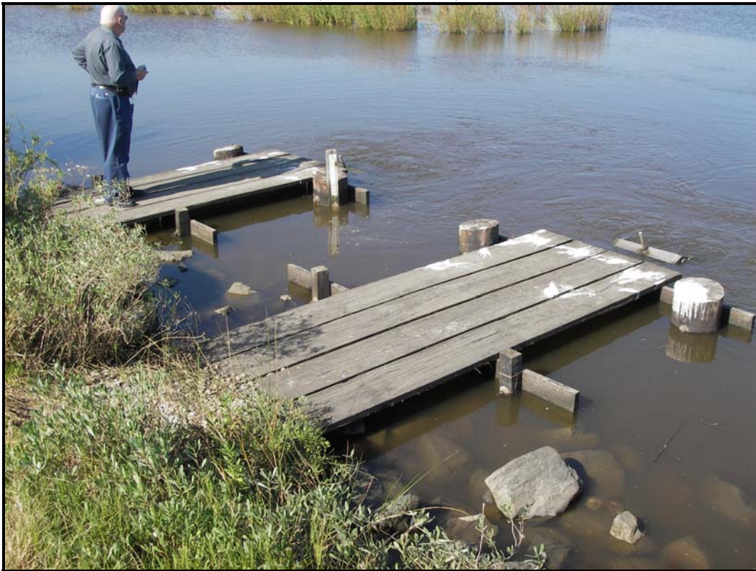
Photo No. 5, Structure No. 12, outlet side.
