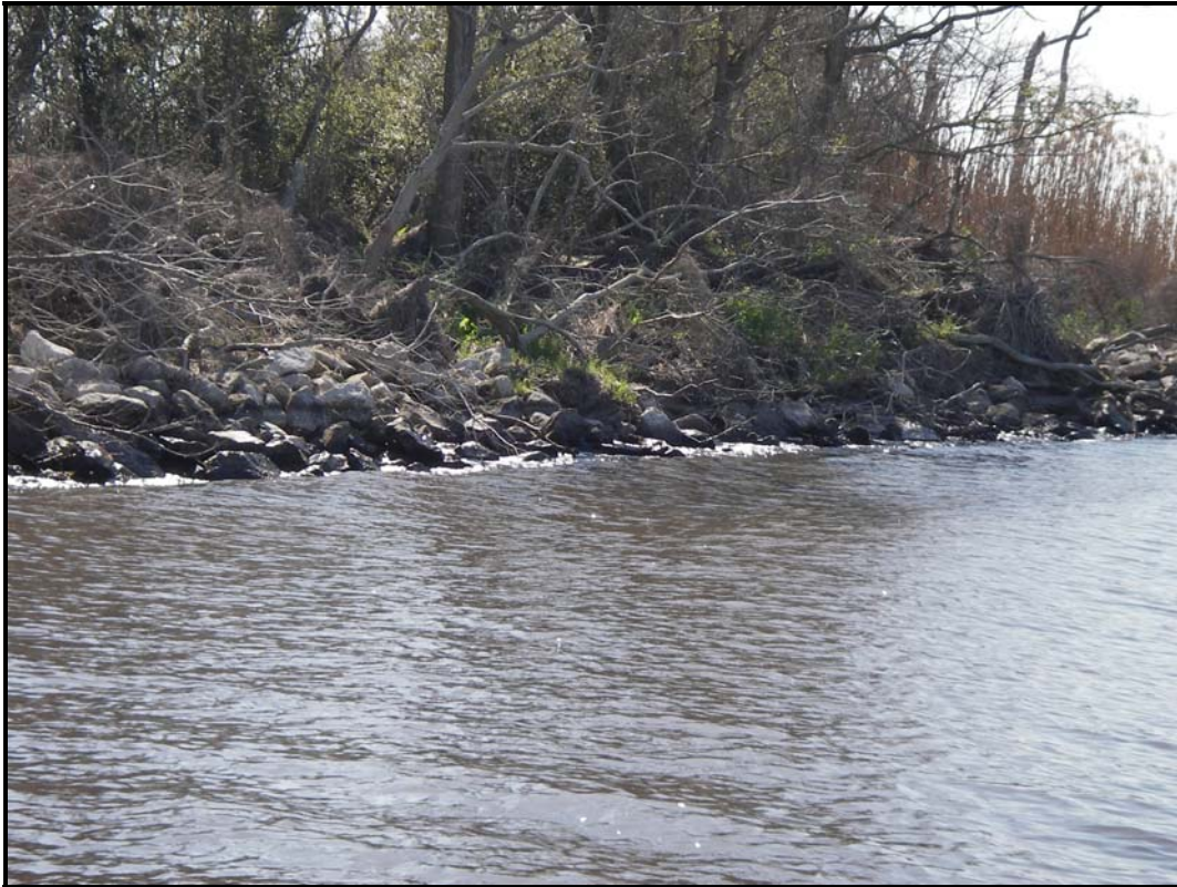
Photo 1 —southern tie-in on Burton Sutton Canal
