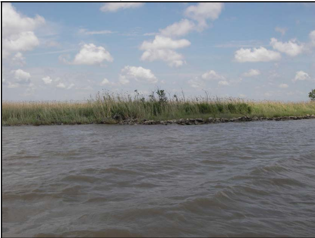
Photo 2 , southern end of rock dike tie-in
