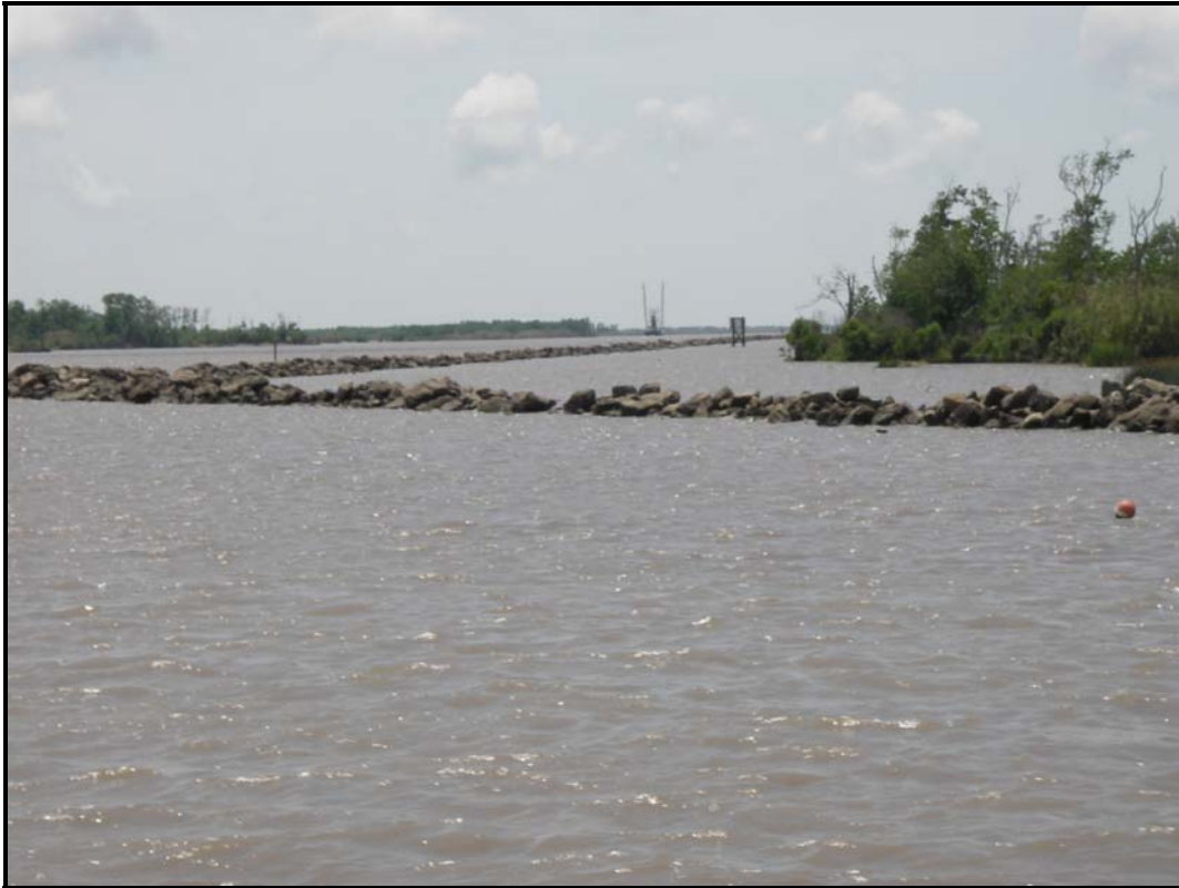
Photo 1 , northern end of rock dike tie-in
