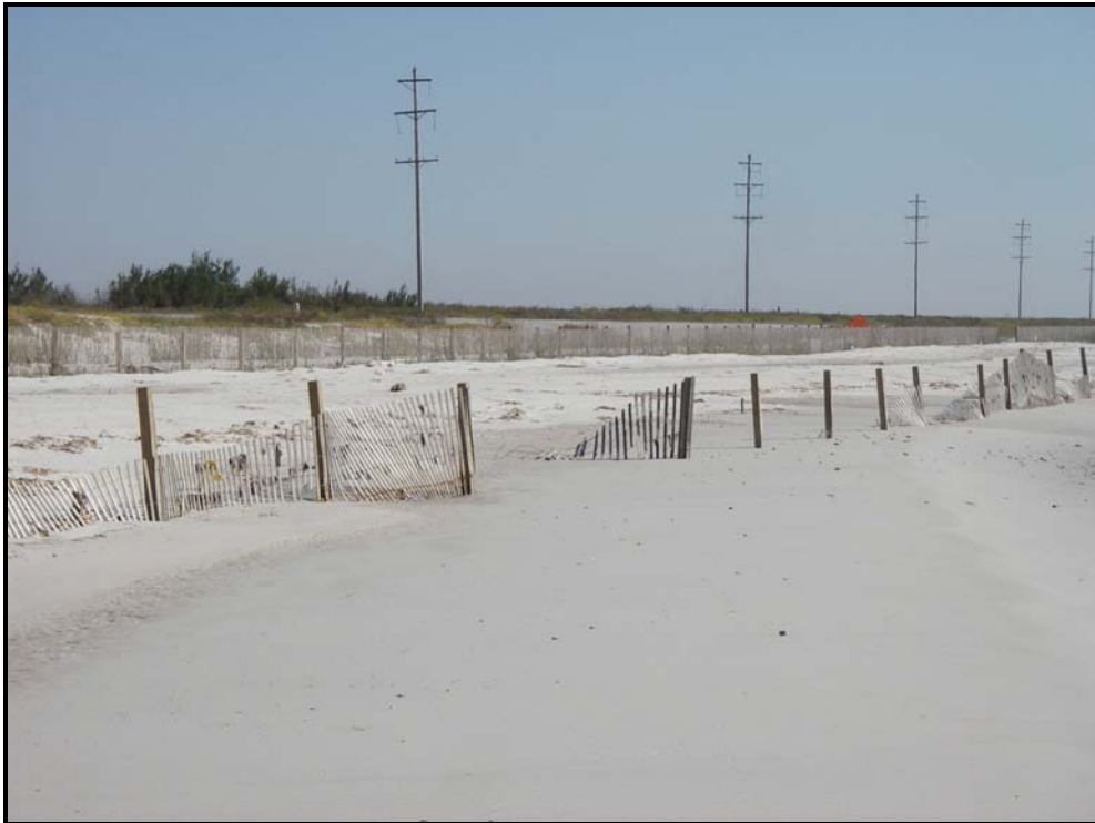
Photo 5, Close up view of damaged secondary fence looking eastward. (10-30-2007)
