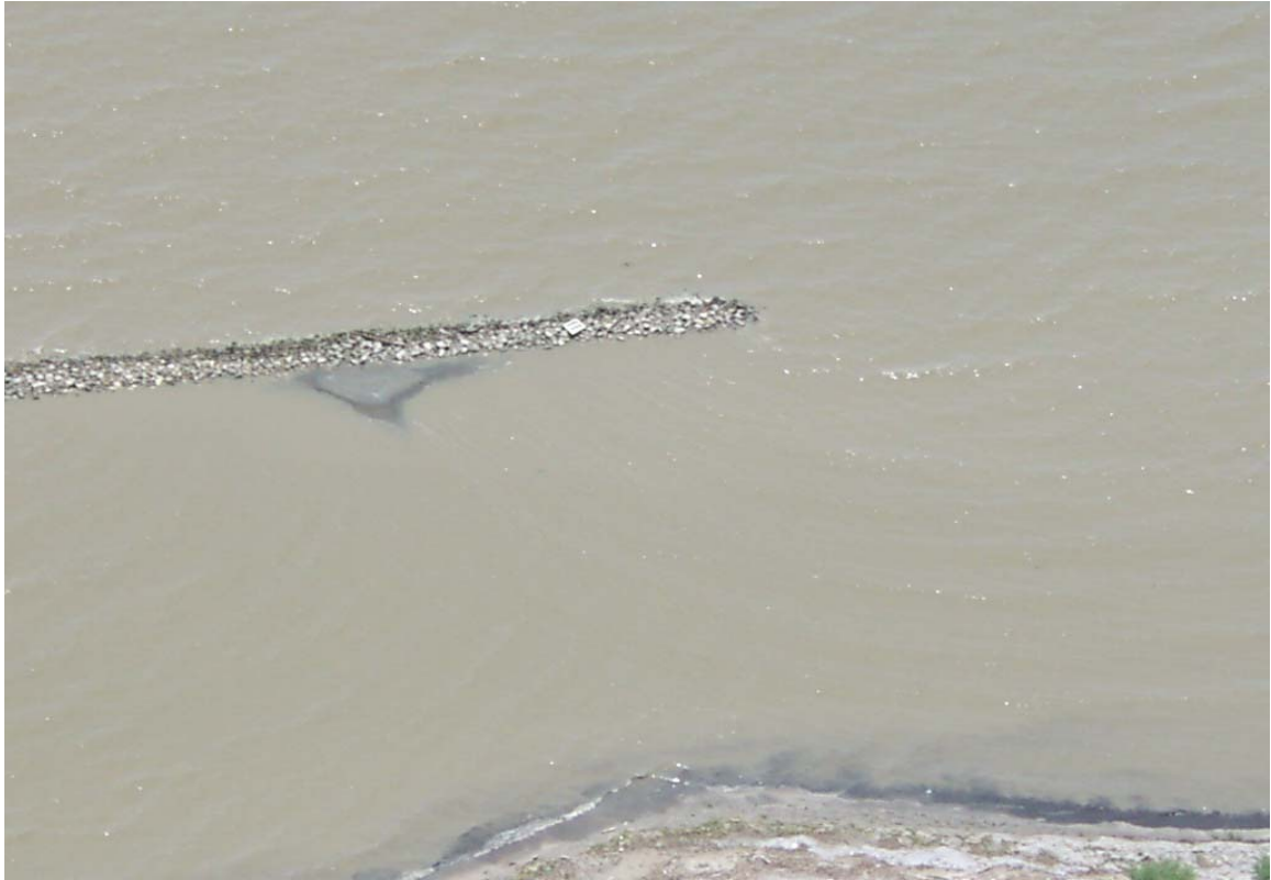
Figure 8. Close-up illustration of sediment accretion behind one of the rock breakwater segments.
