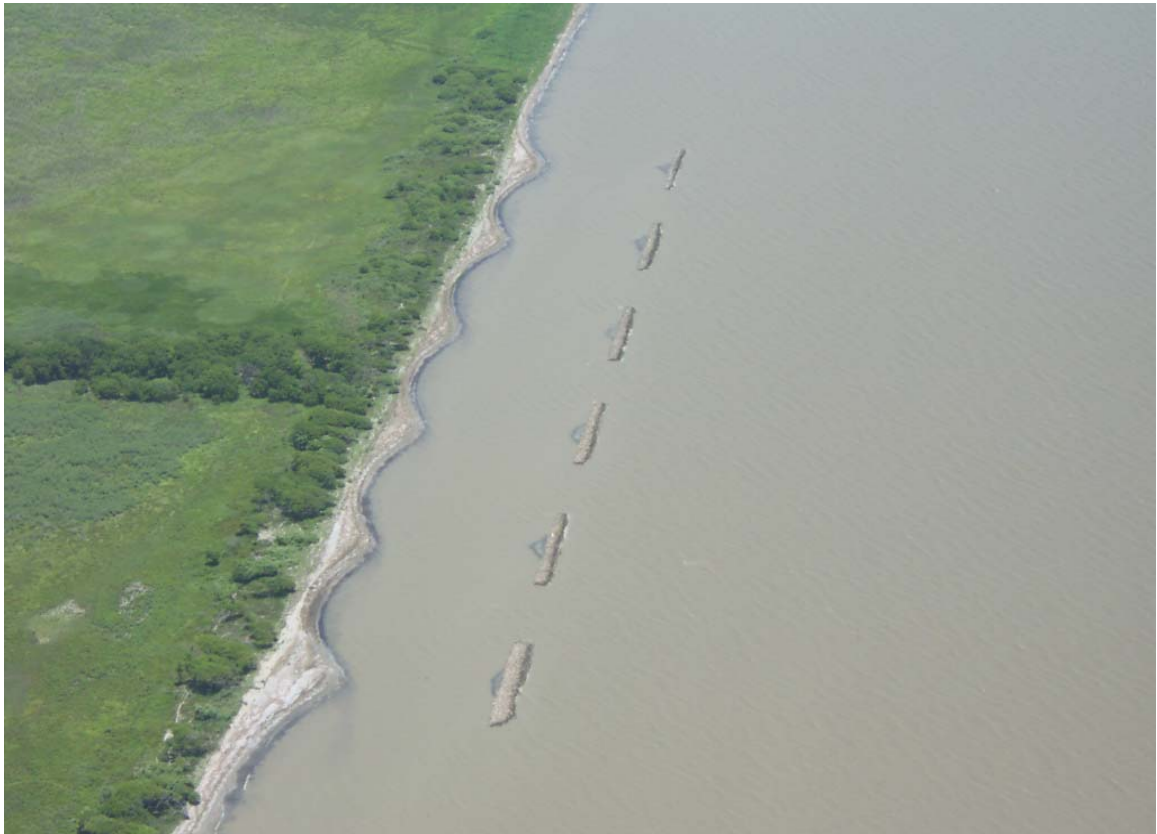
Figure 7. Shoreline of Cheniere au Tigre (aerial view) illustrating sediment accretion behind the rock breakwaters.
