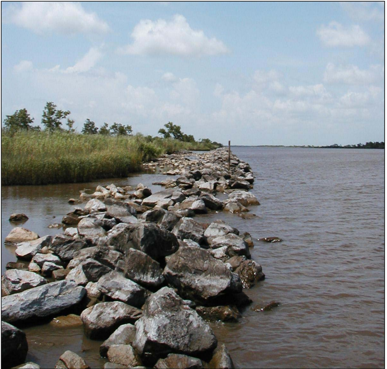
Figure 17. View of the ME-13 rock dike looking north towards station ME13-12 at settlement plate no. 12, taken on July 21, 2003. The dip in the rock dike in front of the settlement plate post will require maintenance to bring this section of dike back up to the specified crown height.
