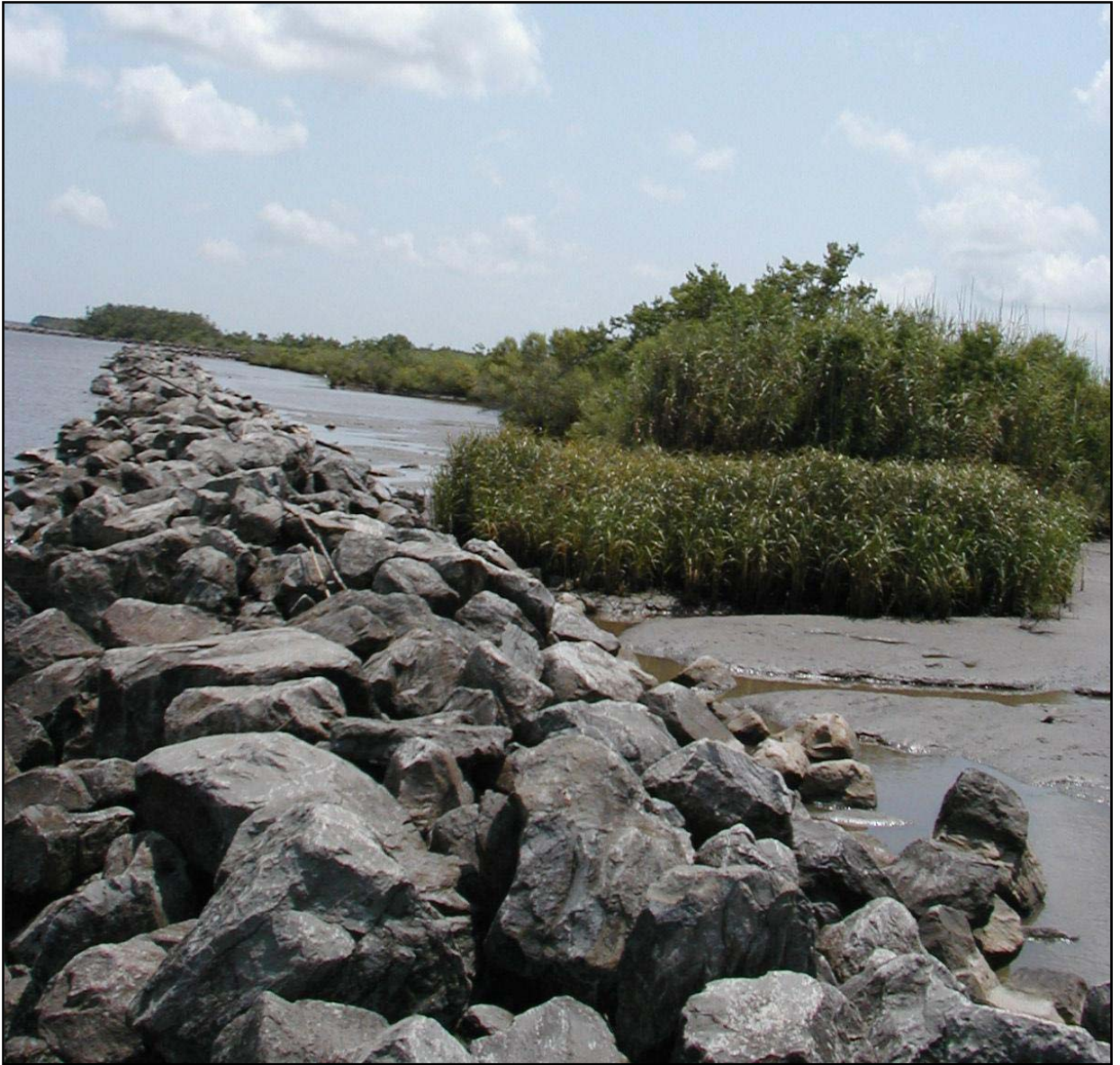
Figure 16. View of the Freshwater Bayou Canal shoreline behind the ME-13 rock dike, looking south from monitoring station ME13-01, as observed on July 21, 2003. Note the healthy condition of the native vegetation along the shoreline and colonizing the shelf of sediment accumulating between the shoreline and rock dike.
