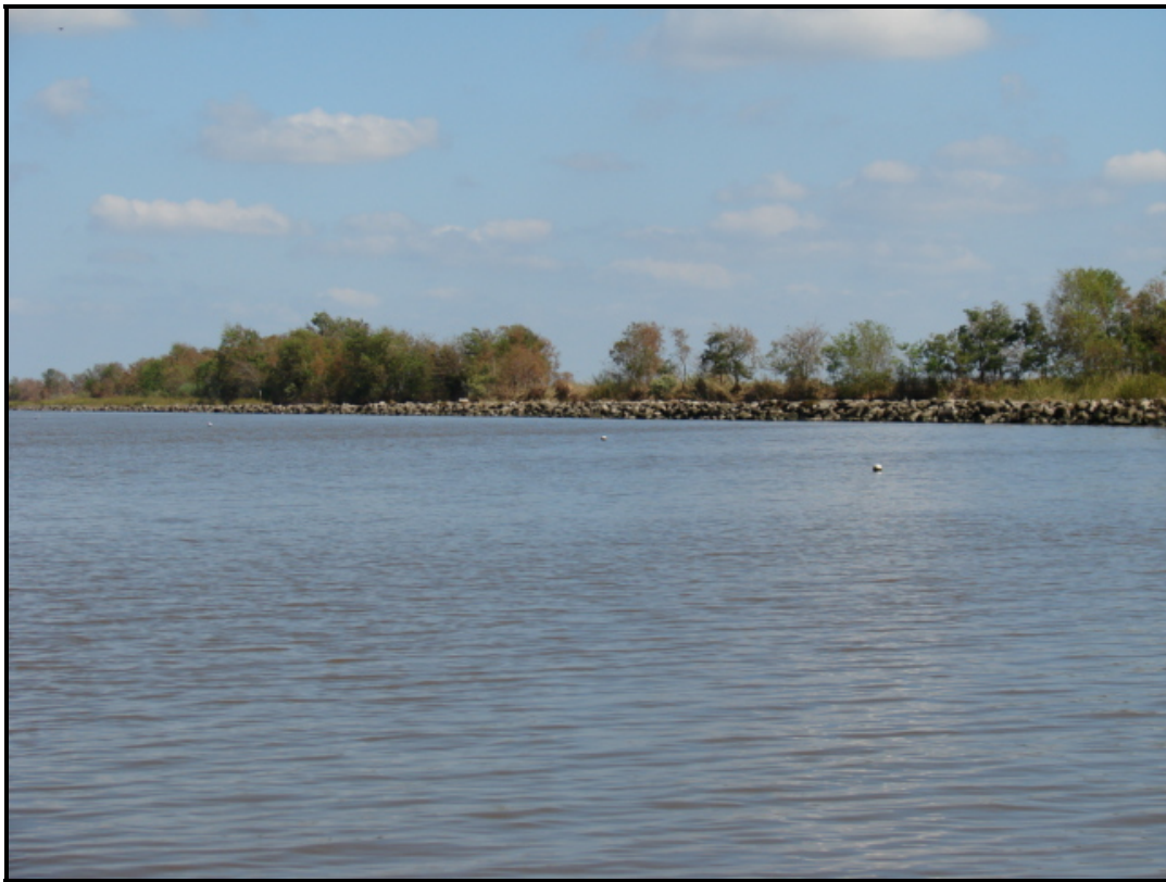
Photo No. 1, Typical rock dike
