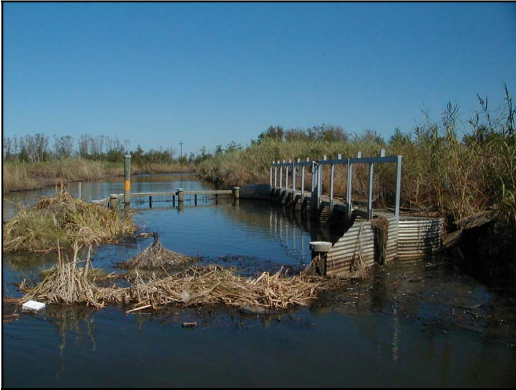
Photo No. 3, Inlet side of structure
