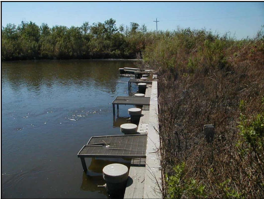
Photo No. 4, Outlet side of structure
