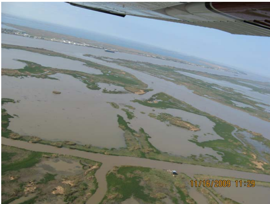
Crevasse No. 81, (view 2) Inside crevasse showing heavy vegetated spoil area and newly deposited sediments.
