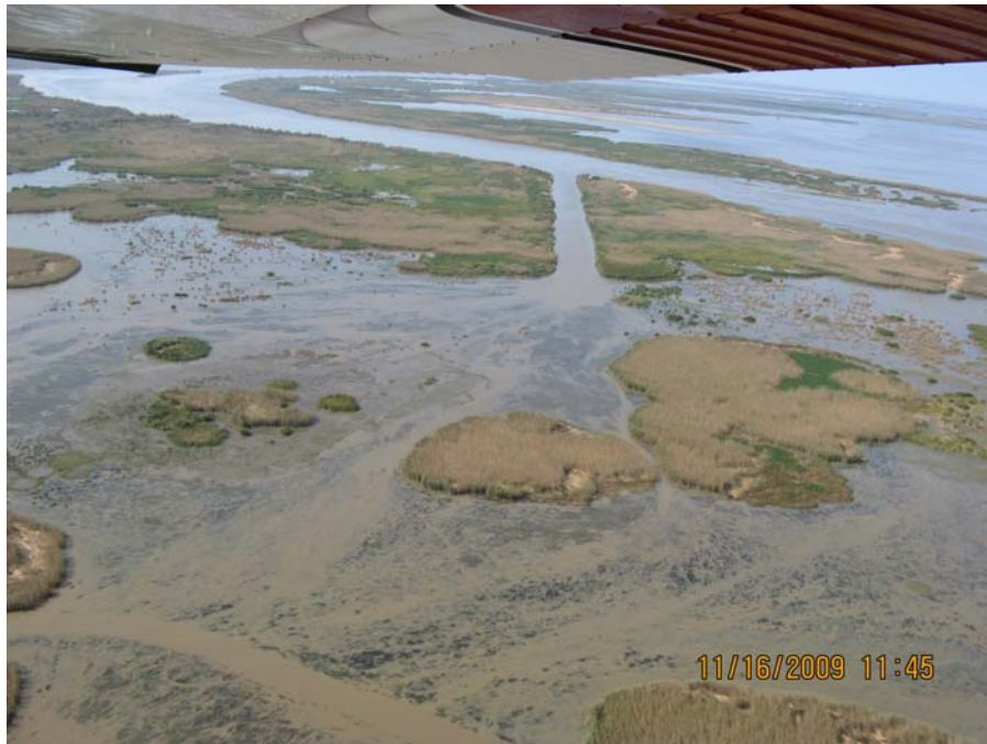
Crevasse No. 11, (view 2) Crevasse end looking at spoil area vegetation and huge amounts of sediments from the pass.
