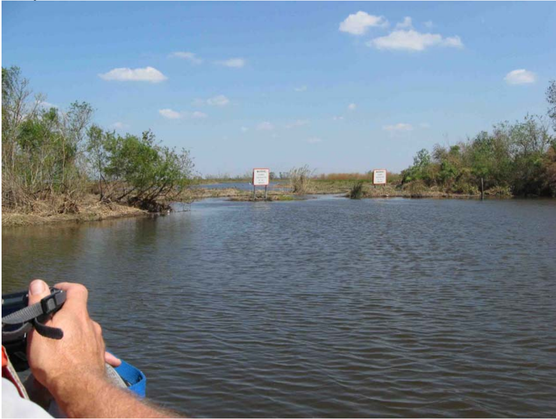
Photo #1 – Structure #14 (Note Gaps)
