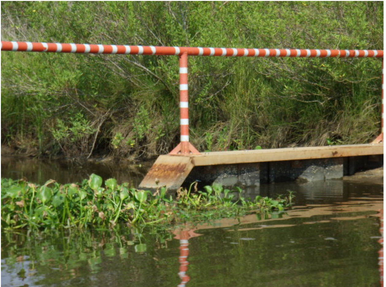
W-14 Weir (Pile Cap, Piles, & Railing)
