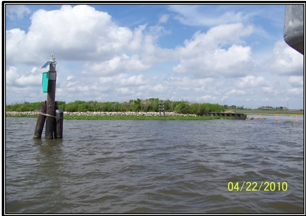
Photo No.50 – view of timber pile dolphin with navigational aid and the bank tie-in on the west side of the Structure No.6.
