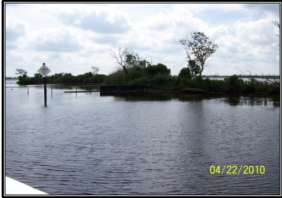
Photo No.21 – view of earthen bank tie-in on the west side of Structure No.24 in Jug Lake. The refurbishment of this earthen embankment tie-in is included in the 2010 Maintenance Project and will be armored with rock riprap approximately 100' west of the structure.
