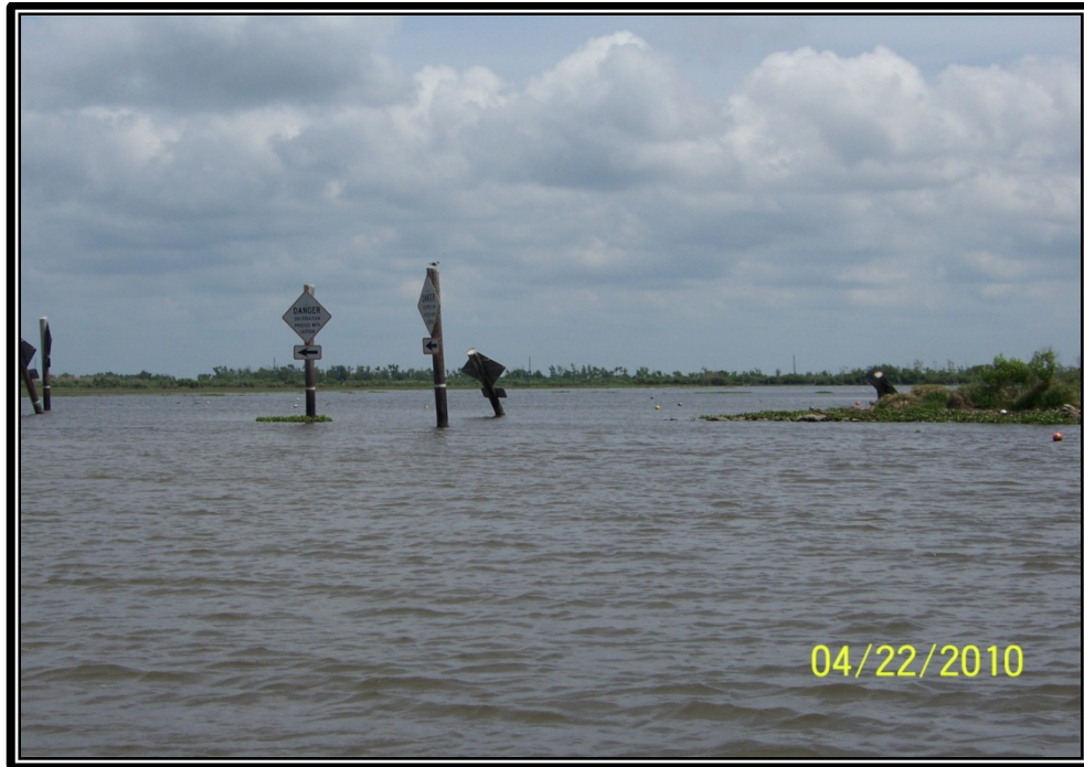
Photo No.53 – view of timber pile warning signs and the southern end of the rock riprap channel liner of Structure No.10. The timber piles that are leaning over were damaged during Hurricane Ike and will be repaired under the 2010 Maintenance Project.
