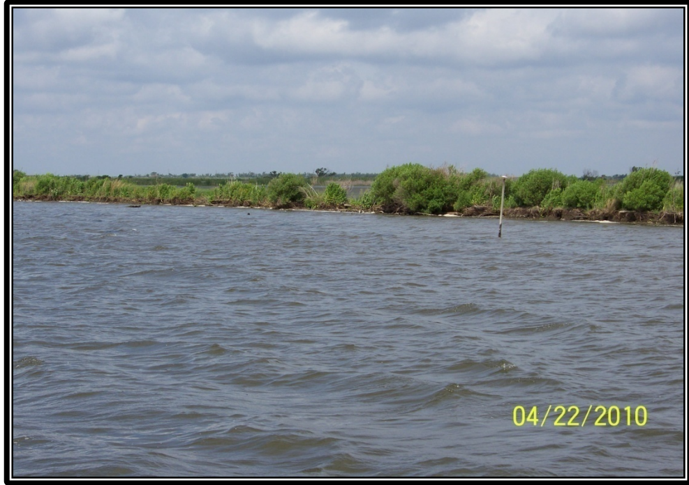
Photo No.33 – view of the bank line and marsh along the north bank of Jug Lake south of Structure No. 21. This section of earthen embankment was reconstructed by the landowner in 2005. This section of bank will be refurbished under the 2010 Maintenance Project.
