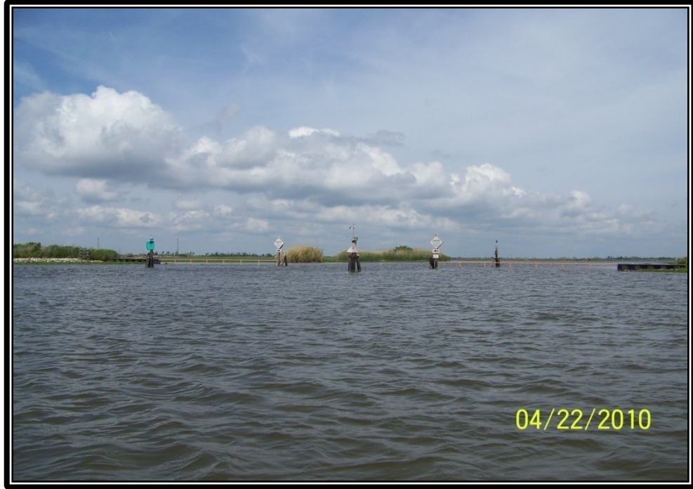
Photo No.49 – view of the fixed crest weir with barge bay and navigational aids at Structure No.6.
