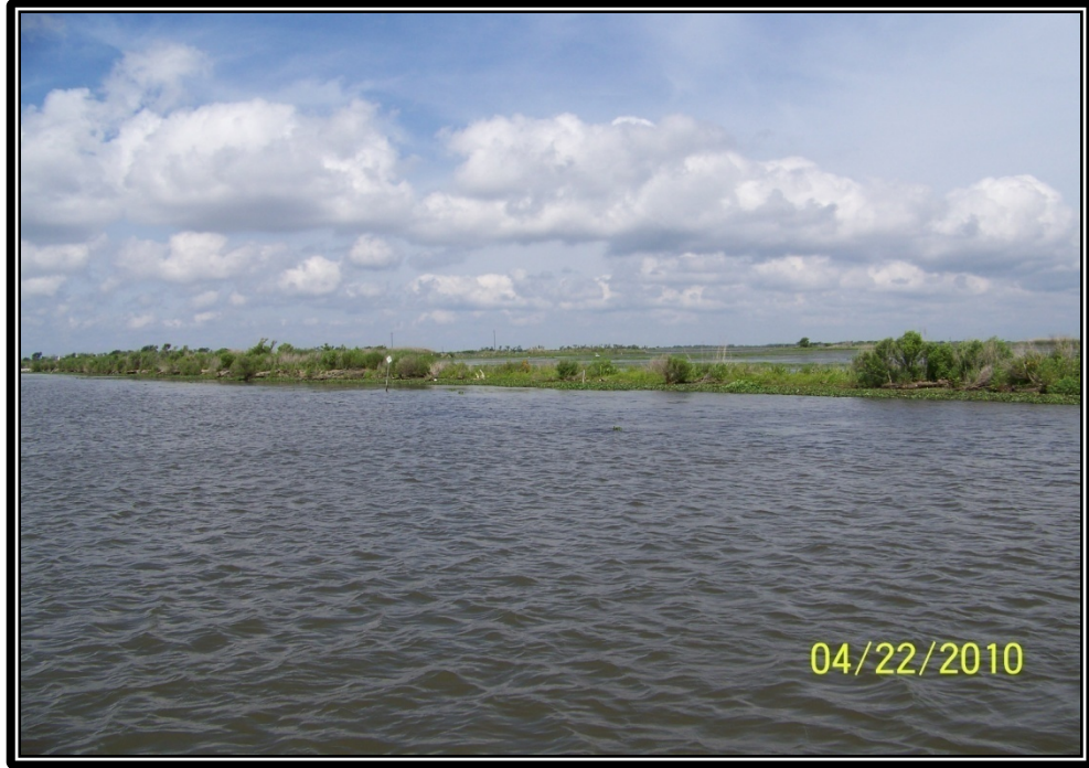
Photo No.47 – view of the existing bank line along the north bank of Jug Lake east of Structure No.6. This bank line appears to be low and will be added to the 2010 Maintenance Project for refurbishment.
