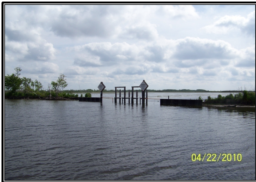
Photo No.24 – view of the two (2) bay variable crest structure (Structure No.23) located in Jug Lake on the northeast side of Jug Lake.
