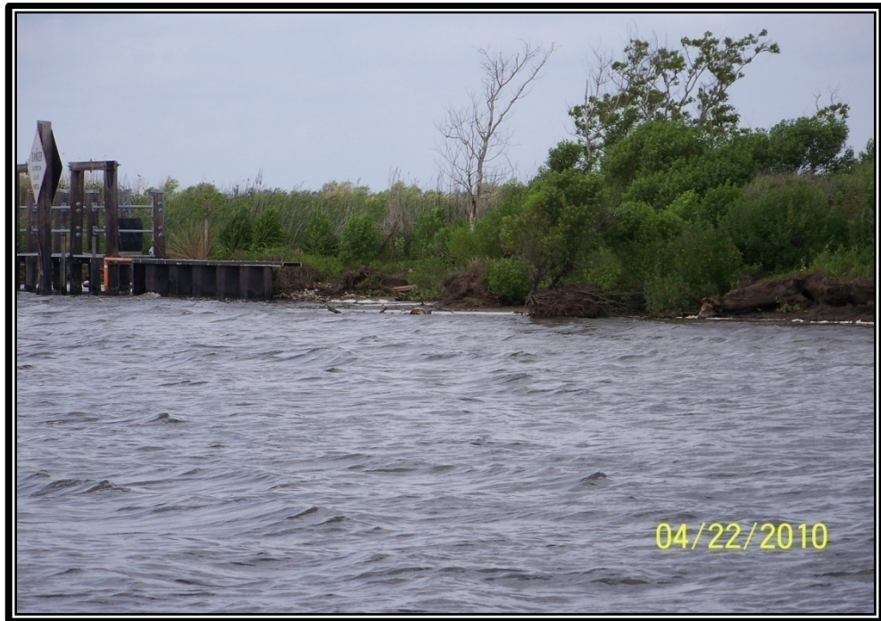
Photo No.28 – view of the exposed steel bulkhead on the northeast side of Structure No. 21 along the north bank of Jug Lake. This embankment will be reconstructed and armored with riprap under the 2010 Maintenance project.
