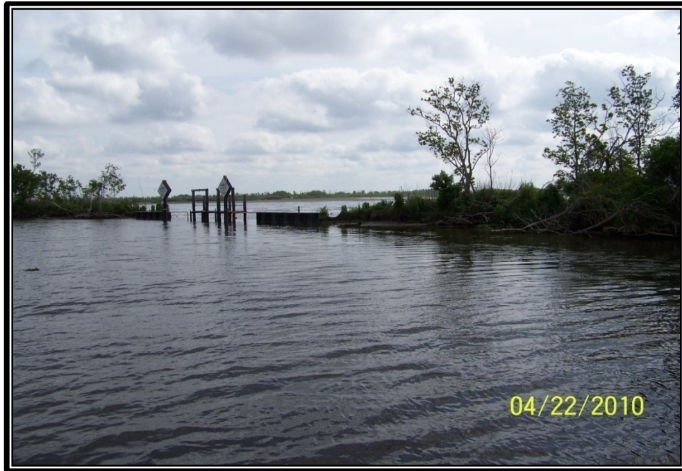
Photo No.23 – view of earthen bank tie-in on the south side of Structure No.23 in Jug Lake. The earthen embankment tie-in is nearly breach on this side with a small amount of material connecting the structure to the embankment. This section of tie-in will be armored with rock riprap approximately 100' south of the structure.
