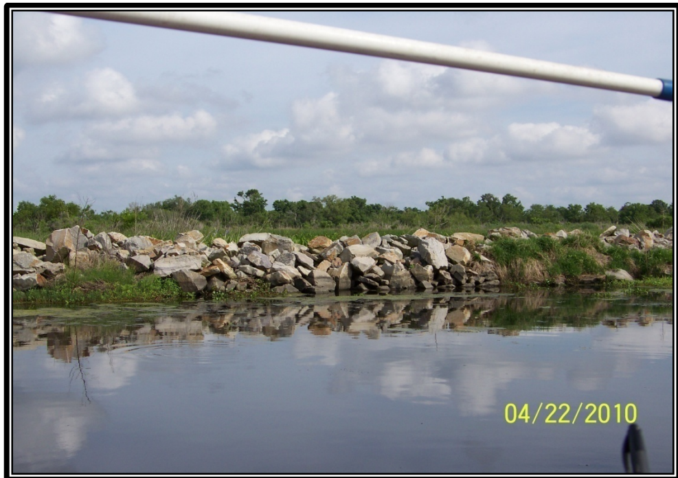
Photo No.2 – rock breach closure “Breach 7” installed in 2003 along an existing location Canal off of Superior Canal looking northeast.
