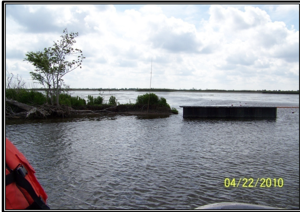
Photo No.25 – view of earthen bank tie-in on the north side of Structure No.23 in Jug Lake. The earthen embankment tie-in is breached on this side. This section of tie-in will be armored with rock riprap approximately 100' north of the structure.
