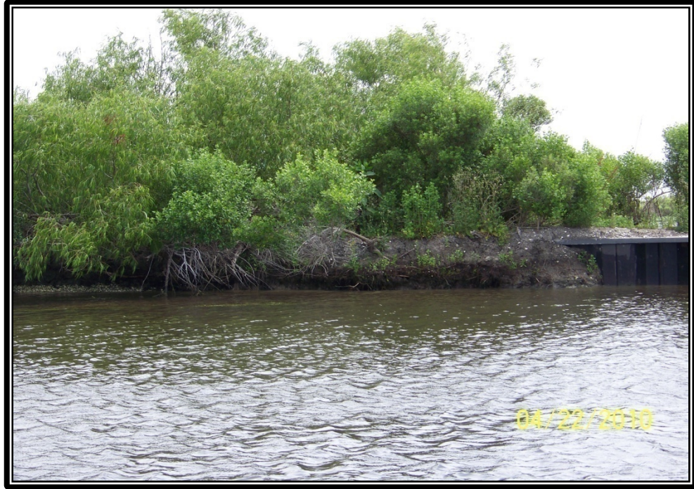
Photo No.57 – view of steel bulkhead and earthen embankment tie-in on the north side of Structure No. 14 along Bayou Carencro.
