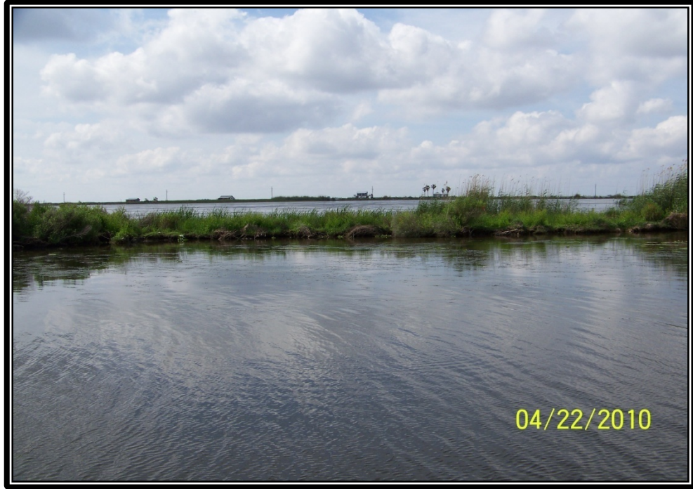
Photo No.17 – view of thin and low bank line along the southern bank of Jug Lake west of Structure No.24. The refurbishment of this bank line is included in the 2010 Maintenance Project.
