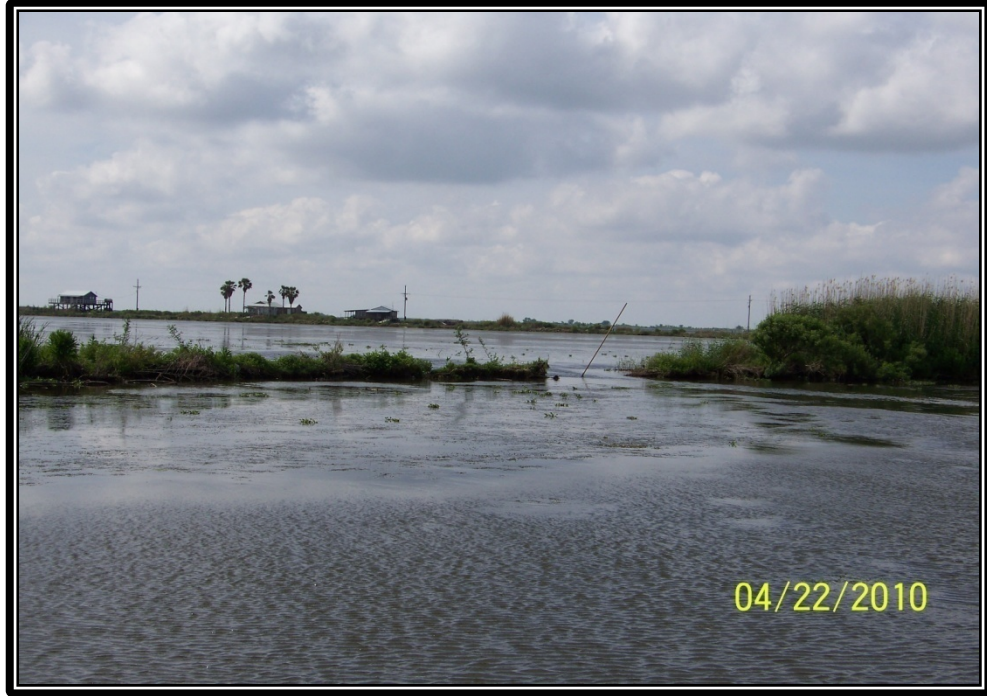
Photo No.15 – view of large breach in the south bank of Jug Lake west of Structure No.24. The breach opened up after Hurricanes Gustave and Ike. The refurbishment of this bank line is included in the 2010 Maintenance Work Plan.
