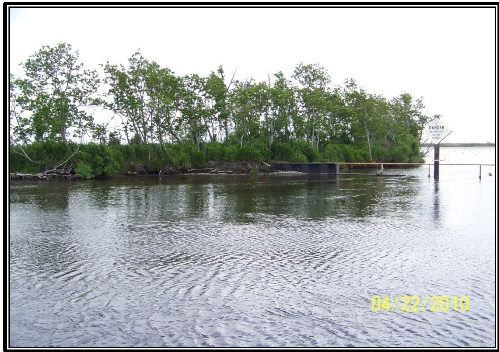
Photo No.22 – view of earthen bank tie-in on the east side of Structure No.24 in Jug Lake. The refurbishment of this earthen embankment tie-in is included in the 2010 Maintenance Project and will be armored with rock riprap approximately 100' east of the structure.
