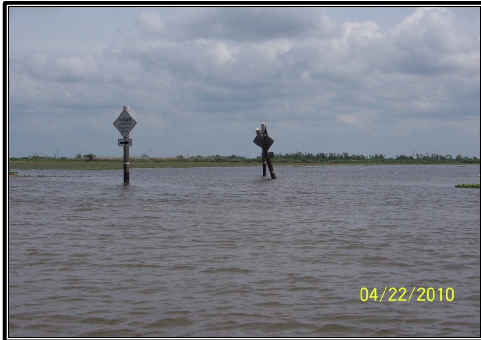
Photo No.54 – view of timber piles, warning signs and the rock riprap channel liner of Structure No.10. The timber piles that are leaning over were damaged during Hurricane Ike and will be repaired under the 2010 Maintenance Project.
