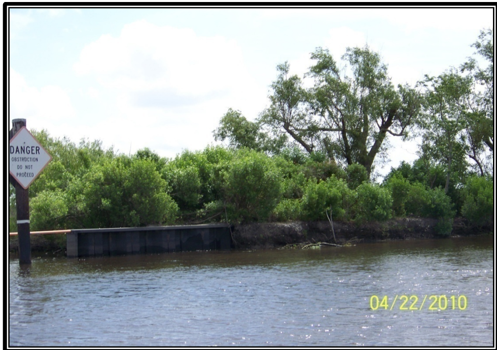
Photo No.56 – view of steel bulkhead and earthen embankment tie-in on the south side of Structure No. 14 along Bayou Carencro.
