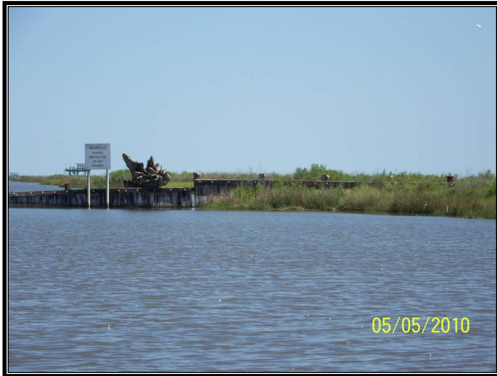
Photo No.11 (3412) – Plug No.6 – view of east tie-in of plug looking north in Transco Canal. A separation in the bulkhead can be noticed to the right of the warning sign.
