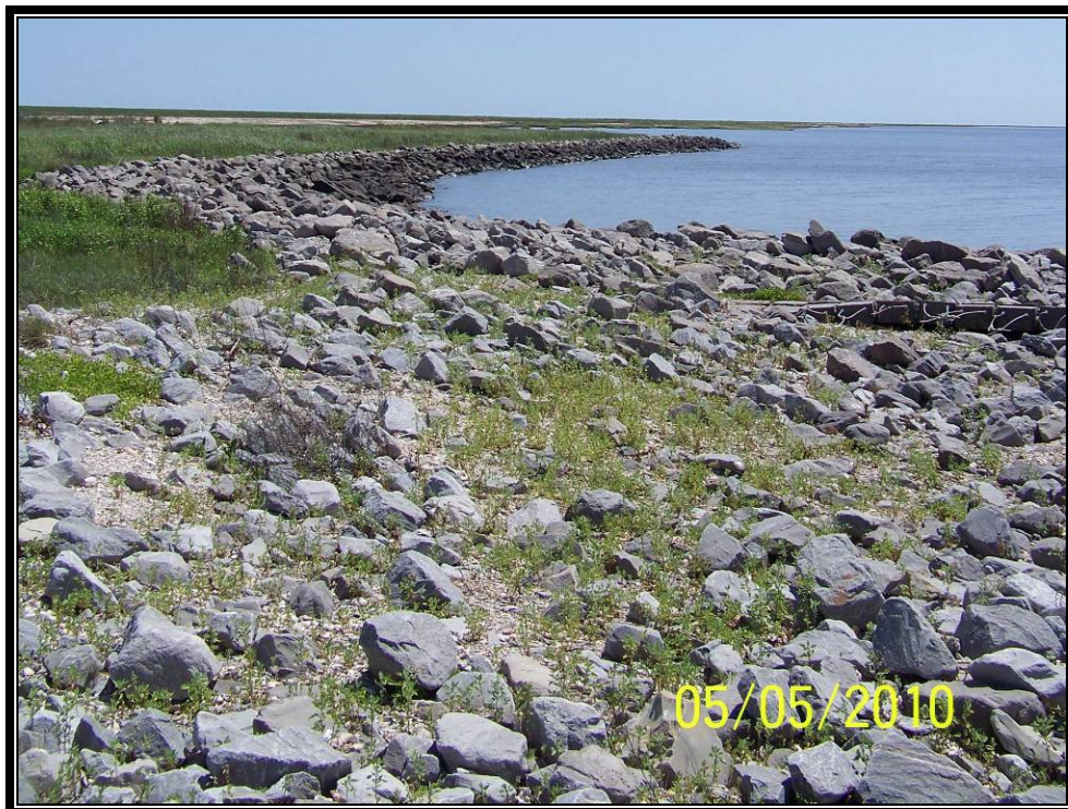
Photo No.6 (3424) – rock covering the existing Petraflex mats on the east side of Plug No. 4A. The rock installed by the pipeline company has been displaced along the shoreline.
