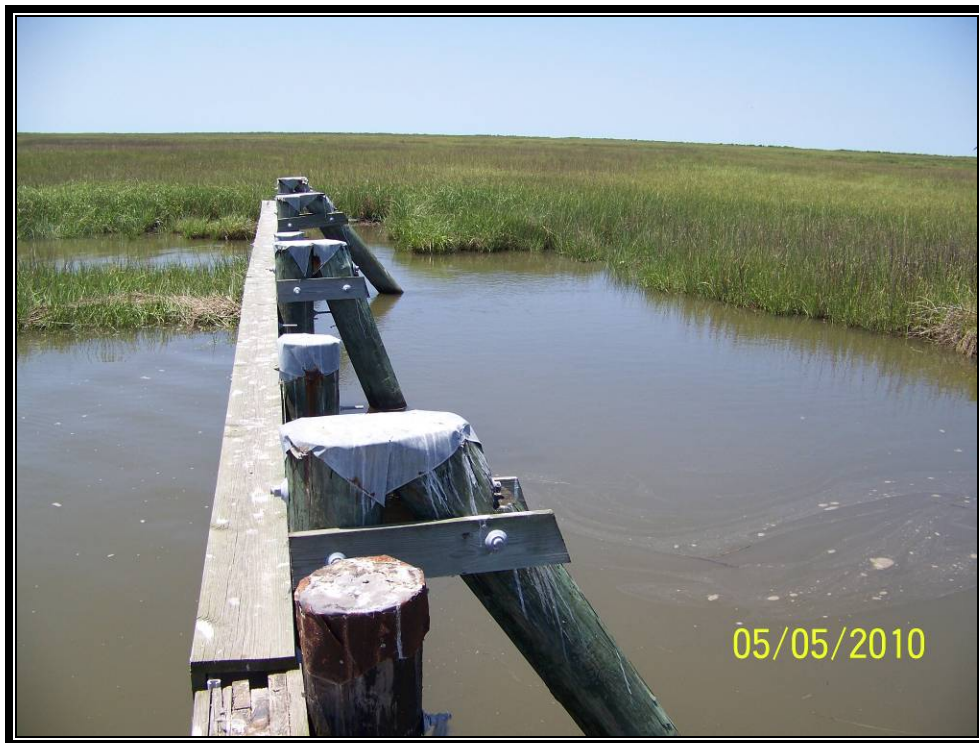
Photo No.20 (3433) – Plug No.8 – View of south tie-in of 2005 maintenance extension of sheet pile wall. Scour has occurred on the southern end of the structure.
