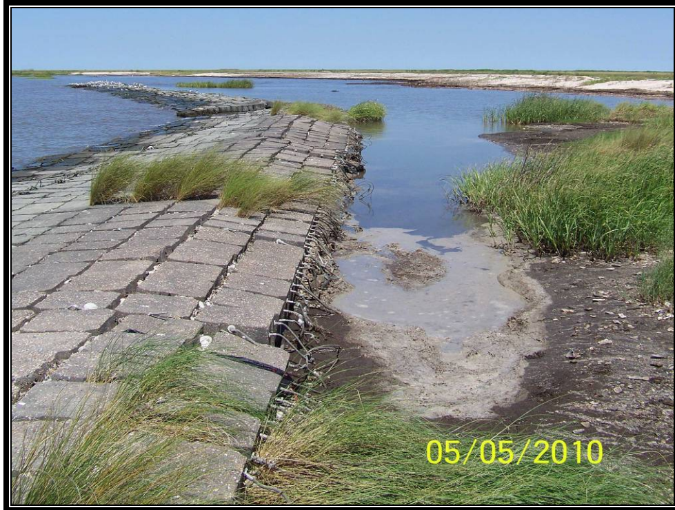
Photo No.3 (3422) – view of Petraflex mats on the west side of Plug No. 4A looking west along the shoreline. The shoreline has retreated as a result of erosion around the mats.
