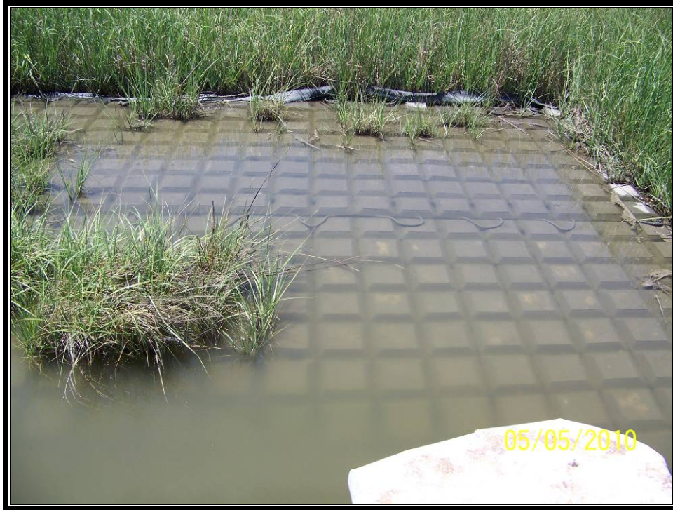
Photo No.21 (3434) - Plug No.8 – view of the Submar scour mats on the southern end of the vinyl bulkhead extension constructed under the 2005 maintenance project. Erosion adjacent to the vinyl bulkhead had taken place. Some of the Submar scour mats were missing.
