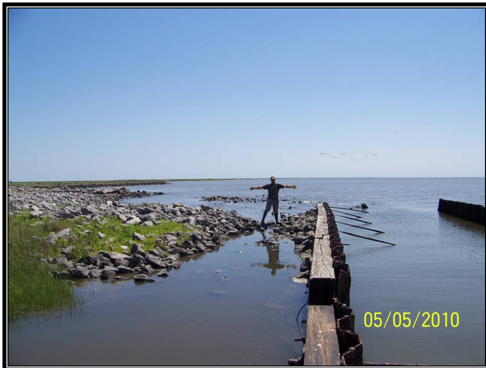
Photo No.4 (3416) – view of Plug No. 4A looking east. The rock material behind the sheet pile placed by the pipeline company has been displaced by recent tropical events.
