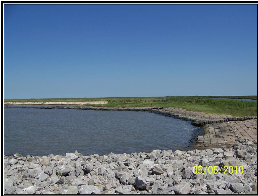
Photo No.2 (3419) – view of marsh behind Petraflex mats on the west side of Plug No. 4A looking east. Erosion can be seen behind the mats.
