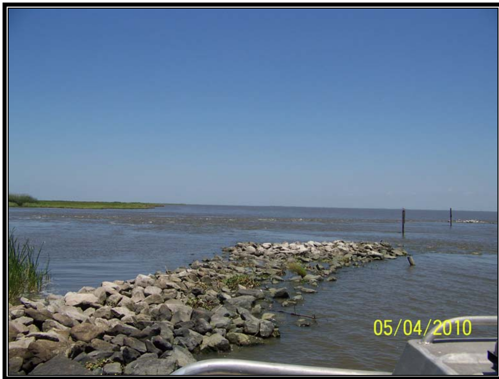
Photo No. 8 - View of breach at northern tie-in of Structure No.3. Photo taken from southern tie-in.
