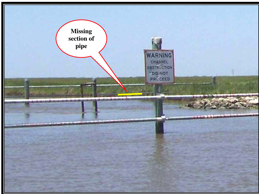
Photo No. 12 – View of the cut pipe in the barricade system at the north tie-in of Structure No. 4.
