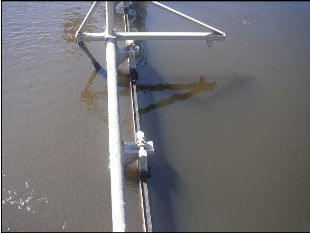
Photo 7 —SRT Gate pillow block on new flap
