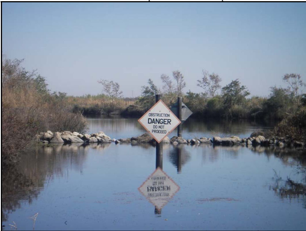
Photo 8 —Rock plug near SRT Gate
