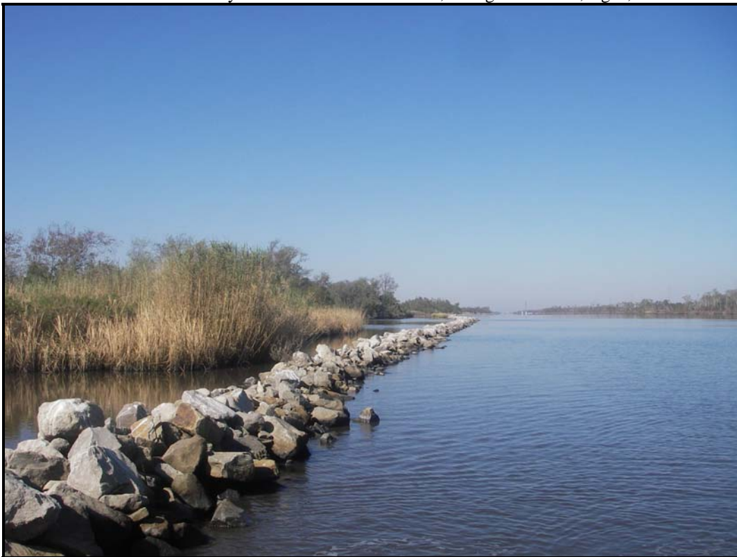
Photo 10 —Typical section of rock dike
