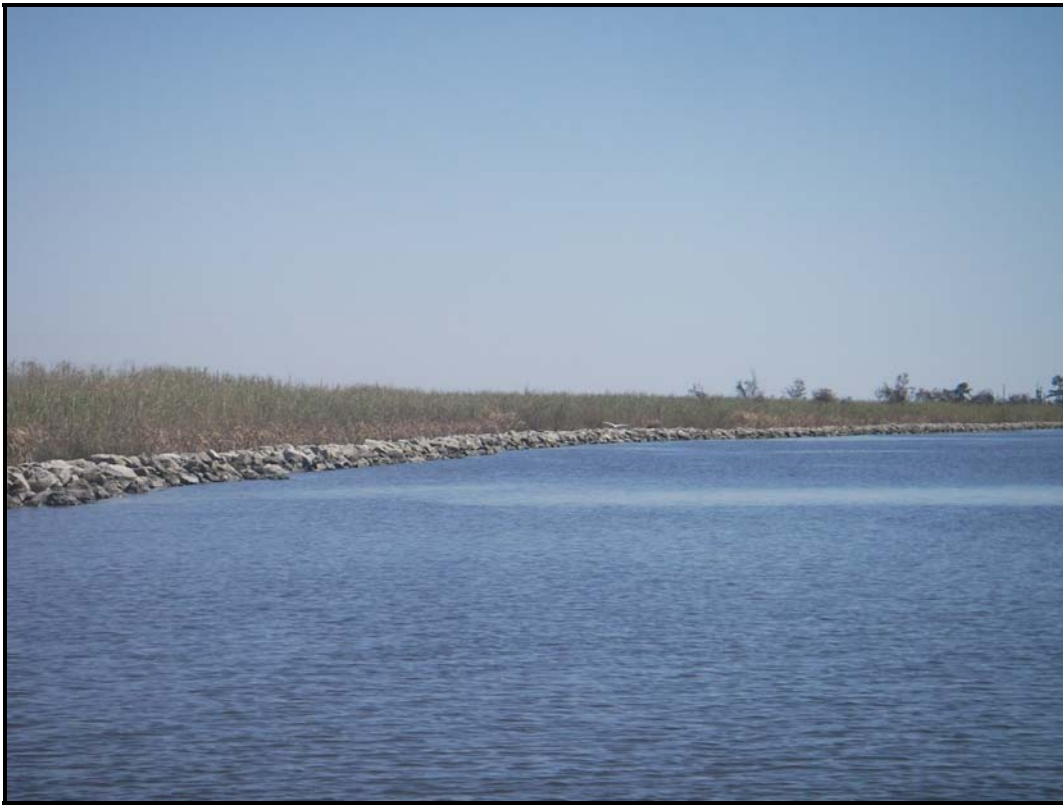
Photo No.1 , Typical rock dike
