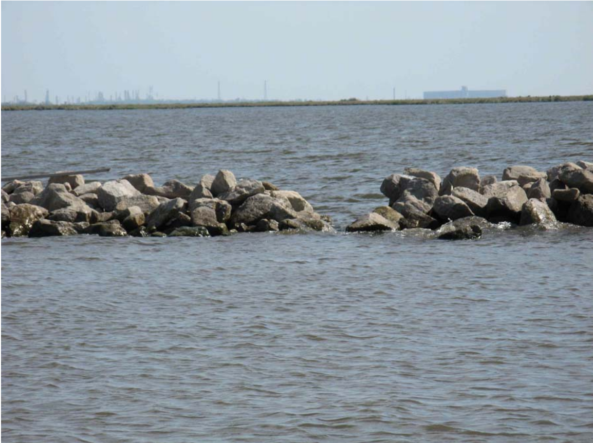
Photo No. 3 – Small gap in Shoreline Protection.
