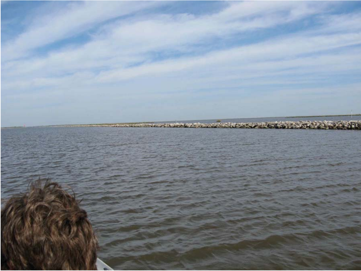
Photo No. 2 – Shoreline Protection.
