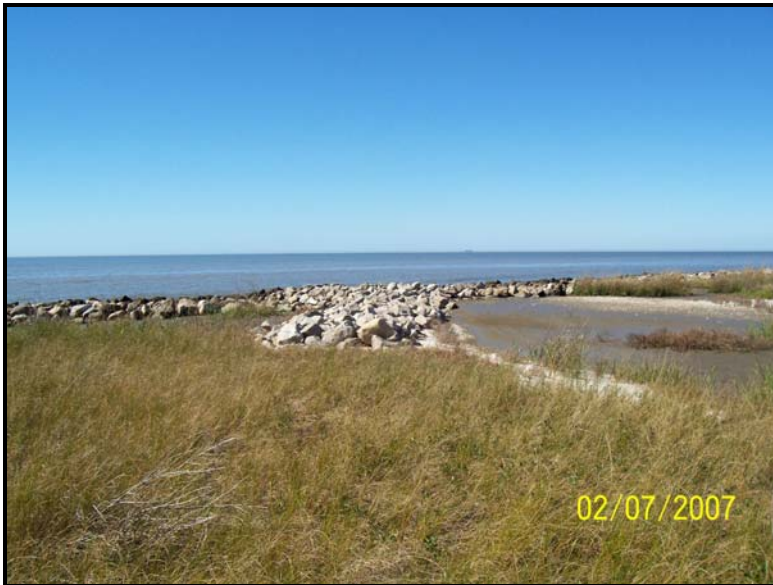
Photo 17. Area 4 Rock Dike – View of 2005 maintenance rock at east end of Area 4 rock dike looking south from shoreline. The rock spur plug extending from the dike can be seen in the foreground.
