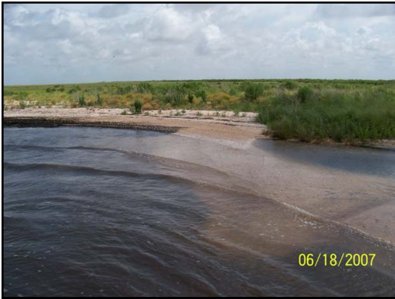
Photo 13. Plug No. 4A – View of continued shoreline erosion behind and beyond west end of the Petraflex mats looking northwest.
