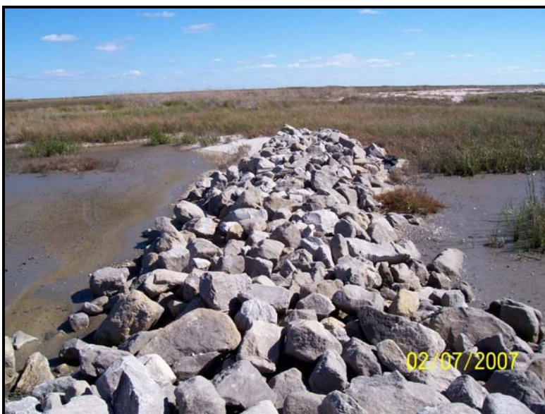
Photo 18. Area 4 Rock Dike – View of rock spur plug extending from dike into marsh. The plug was constructed as part of the 2005 maintenance project.
