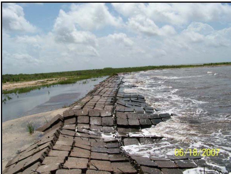
Photo 11. Plug No. 4A – View of Petraflex mats on west side of plug looking east back toward Transco Canal.
