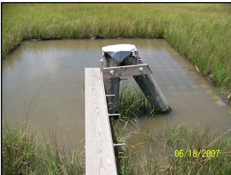
Photo 3. Plug No. 8 – View of south tie-in at end of 2005 maintenance extension of sheet pile wall. Submar mats can be seen submerged. No new scour or erosion of marsh was noted.
