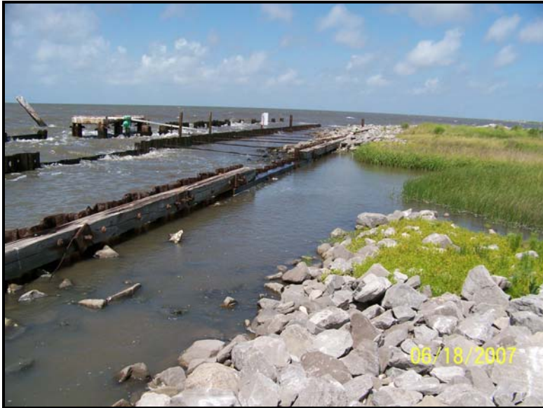
Photo 10. Plug No. 4A – View of steel sheet pile bulkhead at the south end of Transco Canal looking southwest.
