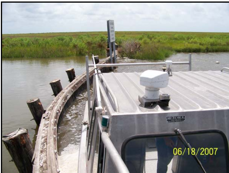
Photo 5. Plug No. 6 – View of plug deflection from approximate centerline of plug looking east in Transco Canal.
