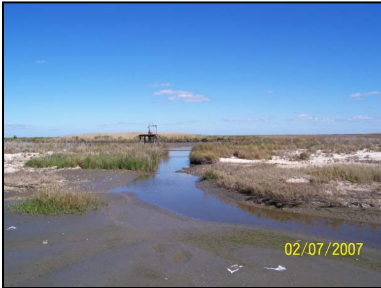
Photo 19. Area 4 Rock Dike – View of breach in Mobil Canal bank behind rock dike. Currently, the spur plug constructed as part of the 2005 maintenance project prevents a direct connection to the Gulf.
