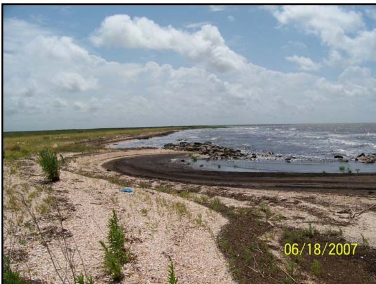
Photo 9. Plug No. 4A – View of east shoreline tie-in of 2005 maintenance rock looking east along shoreline. The small breach resulted from the 2005 hurricanes. Continued shoreline erosion can be seen at the tie-in and beyond.
