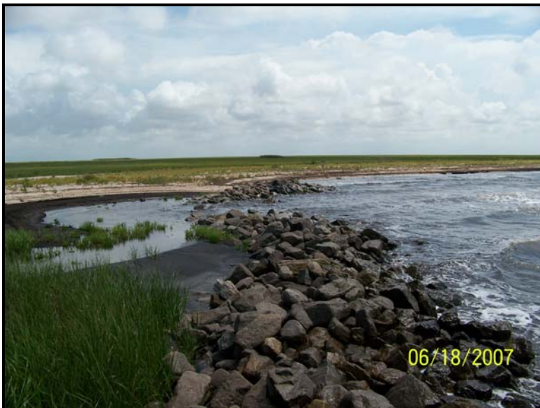
Photo 8. Plug No. 4A – View of east shoreline tie-in of 2005 maintenance rock. The small breach resulted from the 2005 hurricanes. Continued erosion can be seen at the tie-in.
