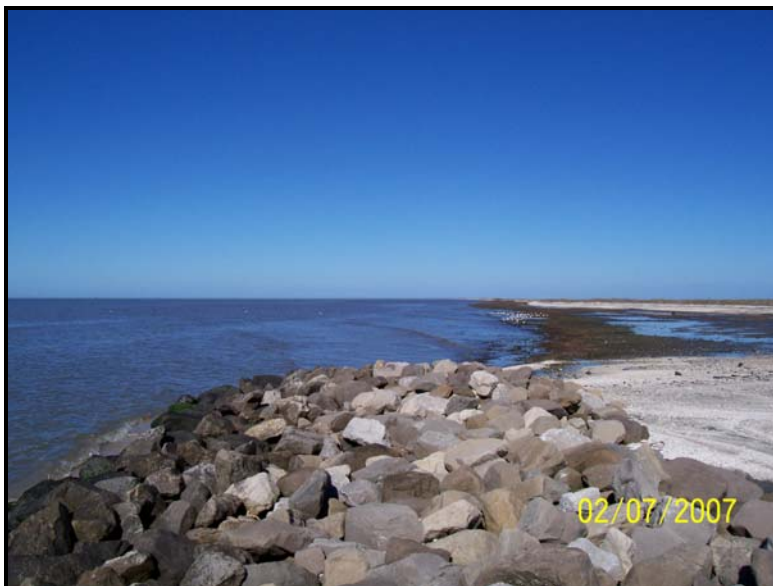
Photo 20. Area 5 Rock Dike – View of west end of rock dike looking northwest. Continued shoreline erosion can be seen just beyond the tie-in.
