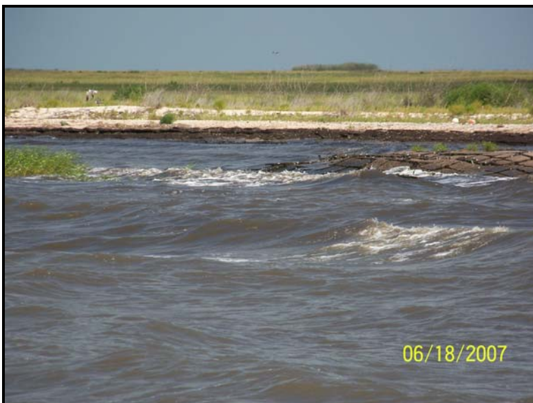
Photo 12. Plug No. 4A – View of west end of Petraflex mats and the continued shoreline erosion at the west tie-in looking northwest.
