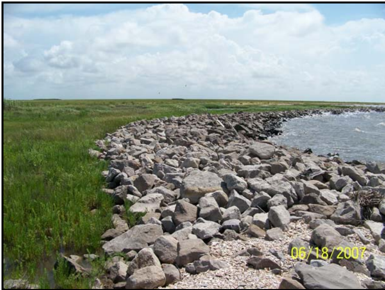
Photo 7. Plug No. 4A – View of east side of plug looking east. This is the additional lift of rock placed over the Petraflex mats as part of the 2005 maintenance project.
