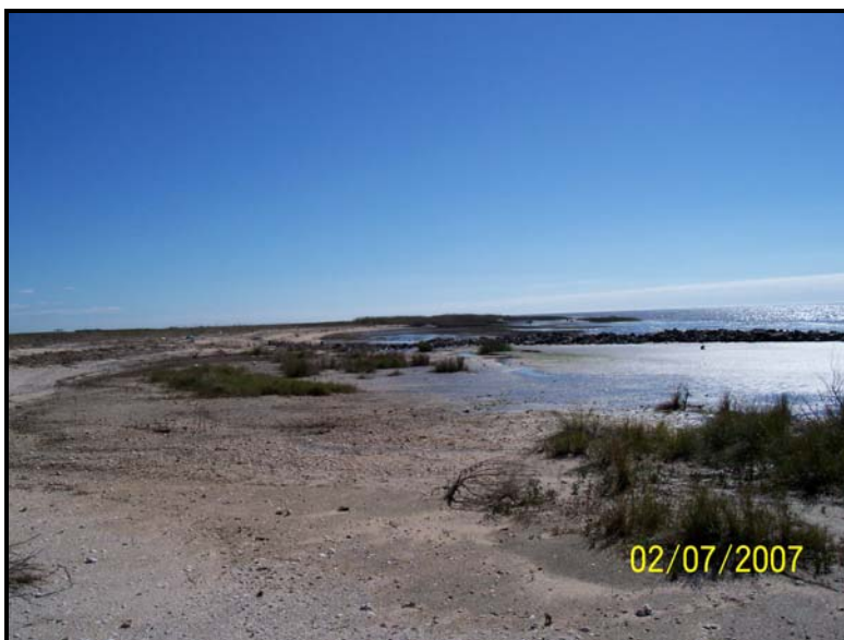
Photo 15. Area 4 Rock Dike – View of east end of 2005 maintenance rock looking southeast from shoreline. Continued shoreline erosion can be seen at tie-in and beyond.
