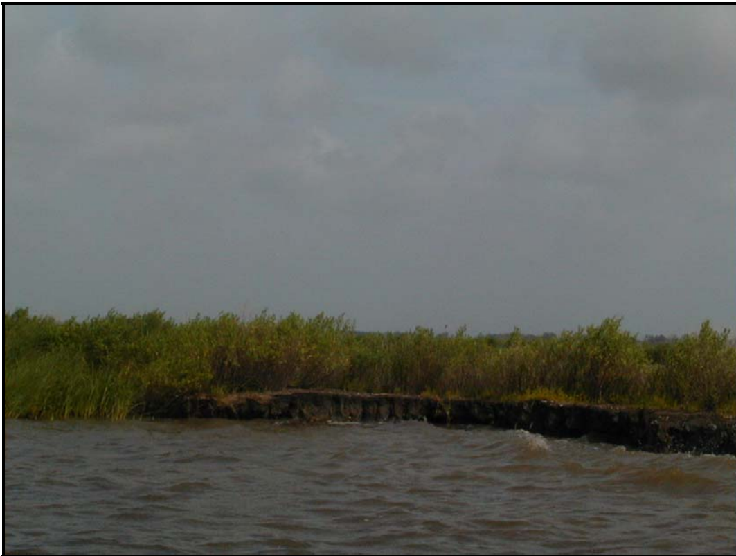
Photo 2, Typical eroded terrace.
