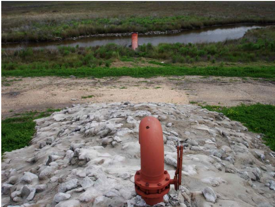
Photo #4 – CTU #5. Pump discharge pipe crossing under levee.
