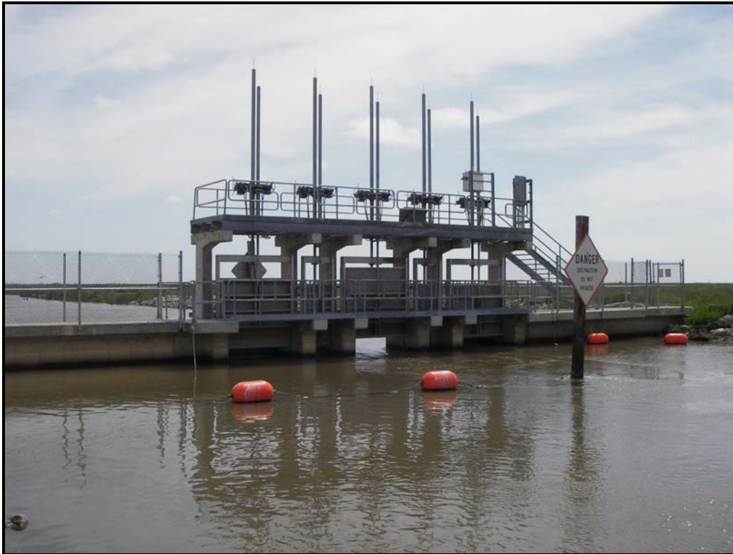
Photo No. 3, Inside view of West Cove Structure. (2007-03-22)
