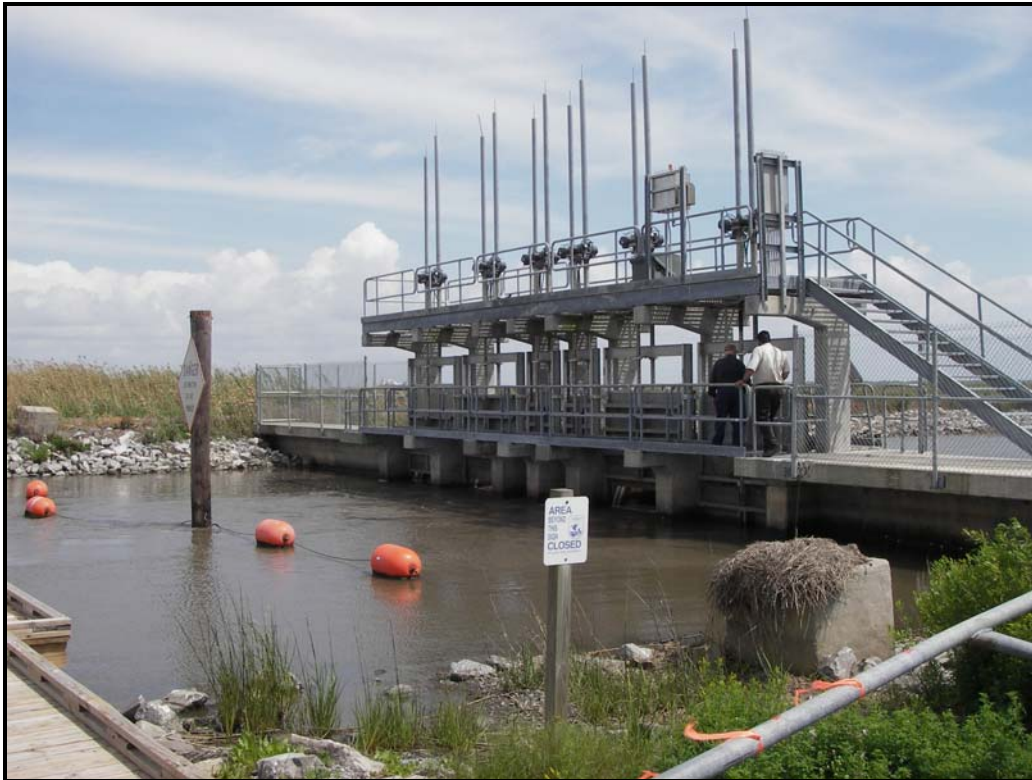
Photo No.1, Inside view of Hog Island Gully Structure. (2007-03-22)
