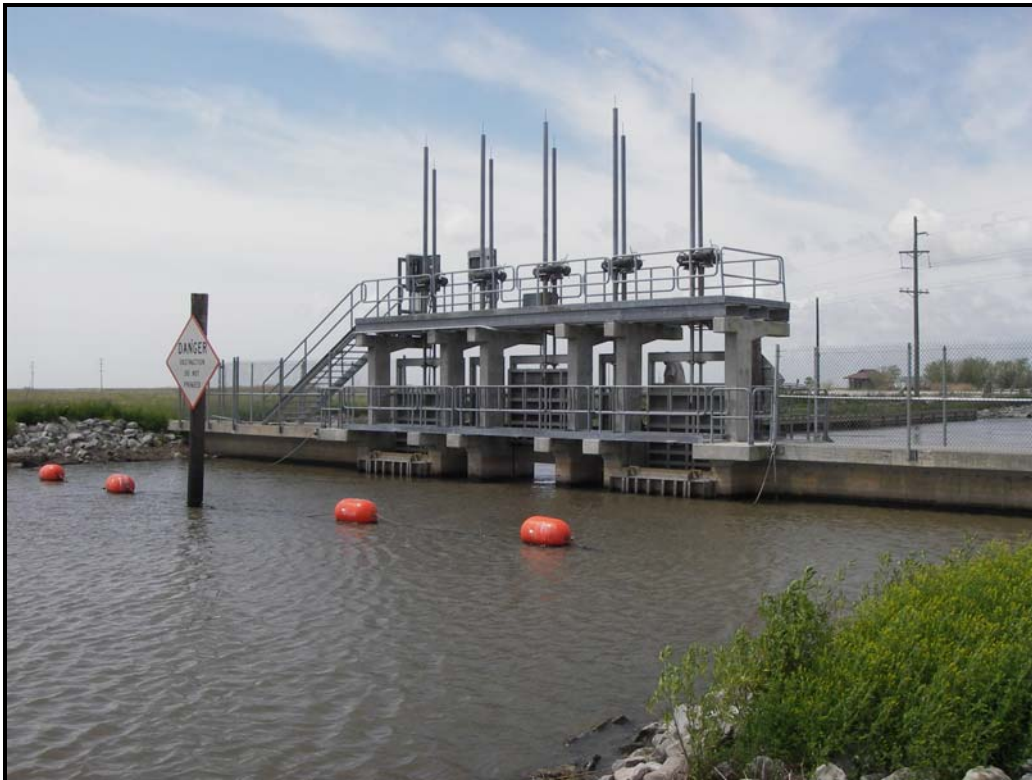
Photo No. 4, Lake side view of West Cove Structure. (2007-03-22)
