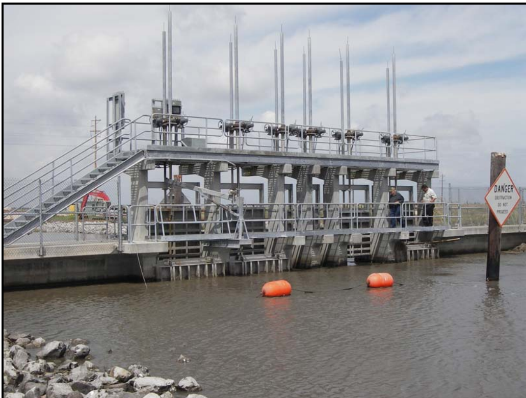
Photo No. 2, Lake side view of Hog Island Gully Structure. (2007-03-22)
