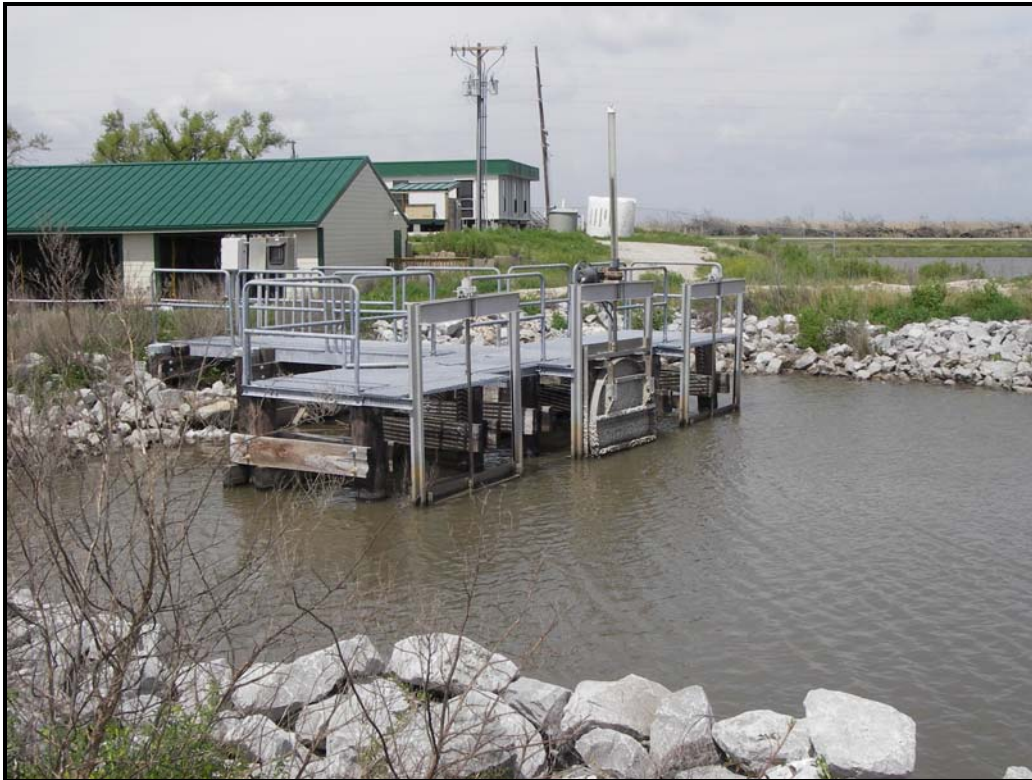
Photo No. 5, Inlet side of Headquarters Structure. (2007-03-22)
