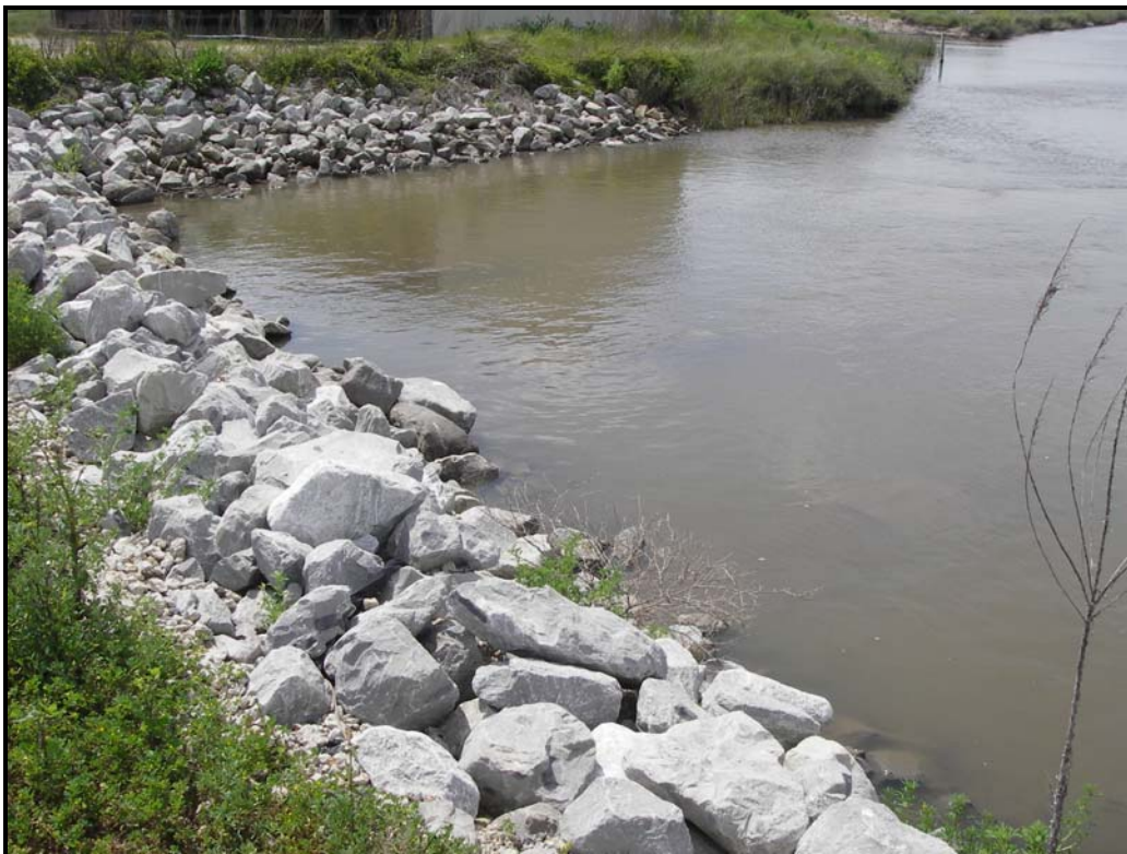
Photo No. 6, Outlet side of Headquarters Structure. (2007-03-22)
