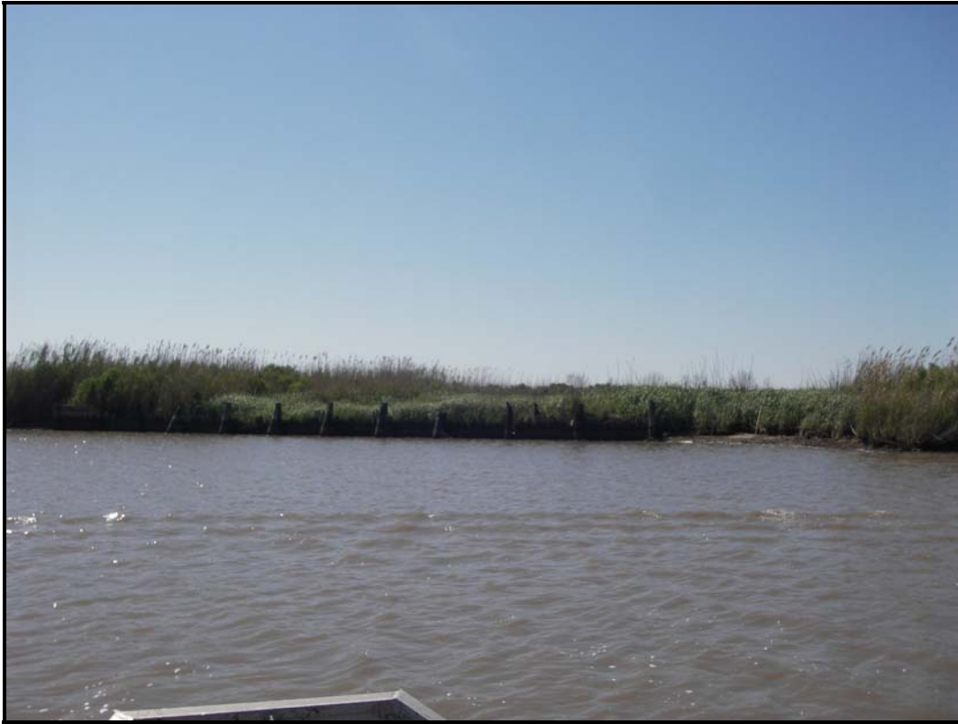
Photo 1, Area 1, View looking south at timber bulkhead.
