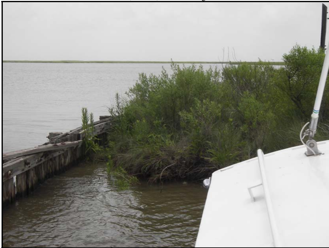
Photo 6, Area 3, near bulkhead on north end.
