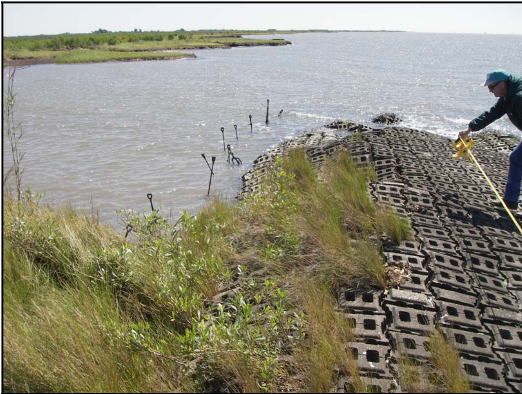
Photo 4, Area 2, East side of concrete mats.
