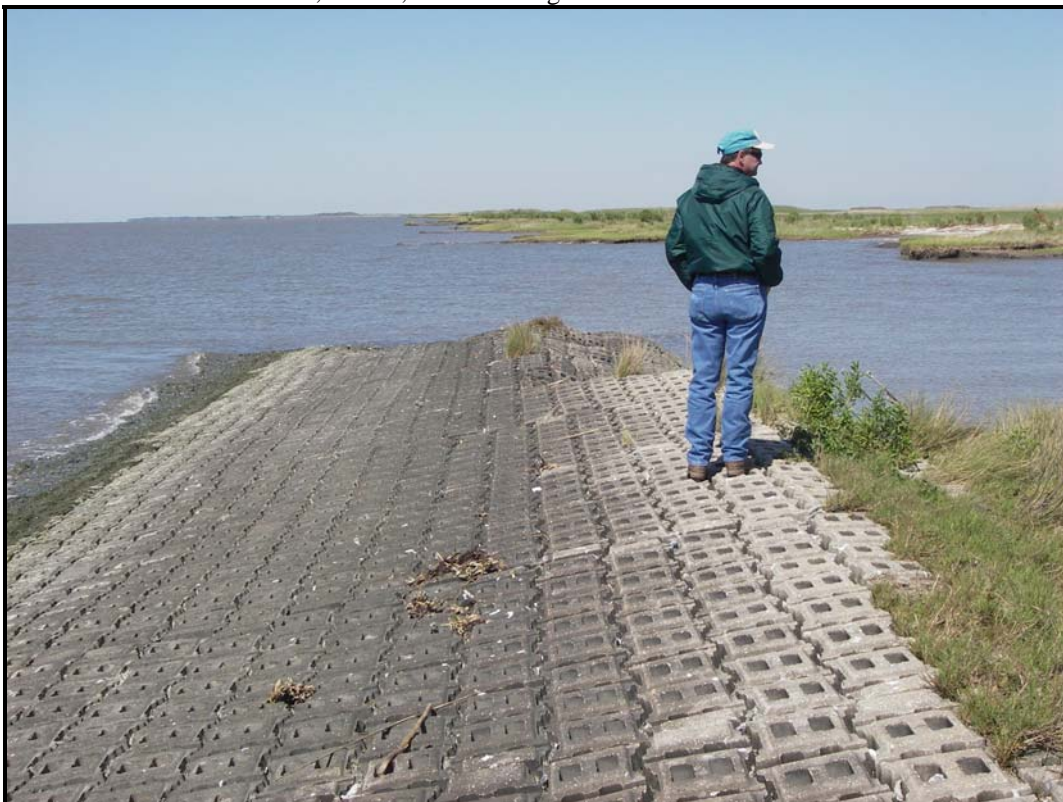
Photo 2, Area 2, West side of concrete mats.
