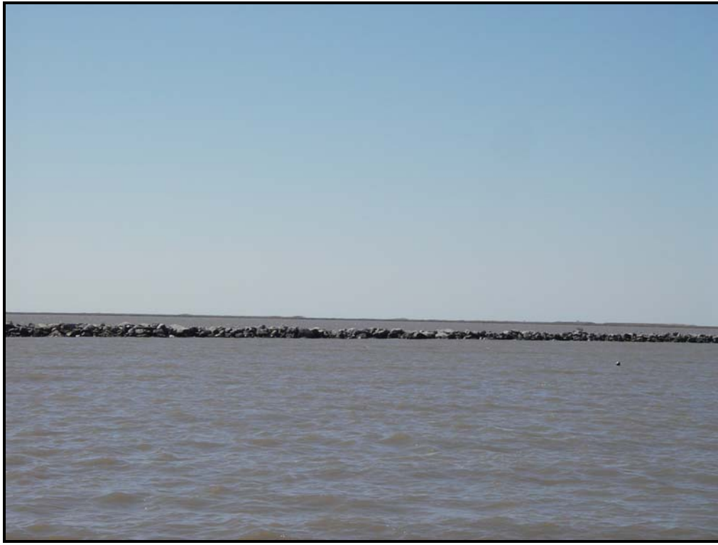
Photo 5, Typical view of Lake Sand Closure No. 4.
