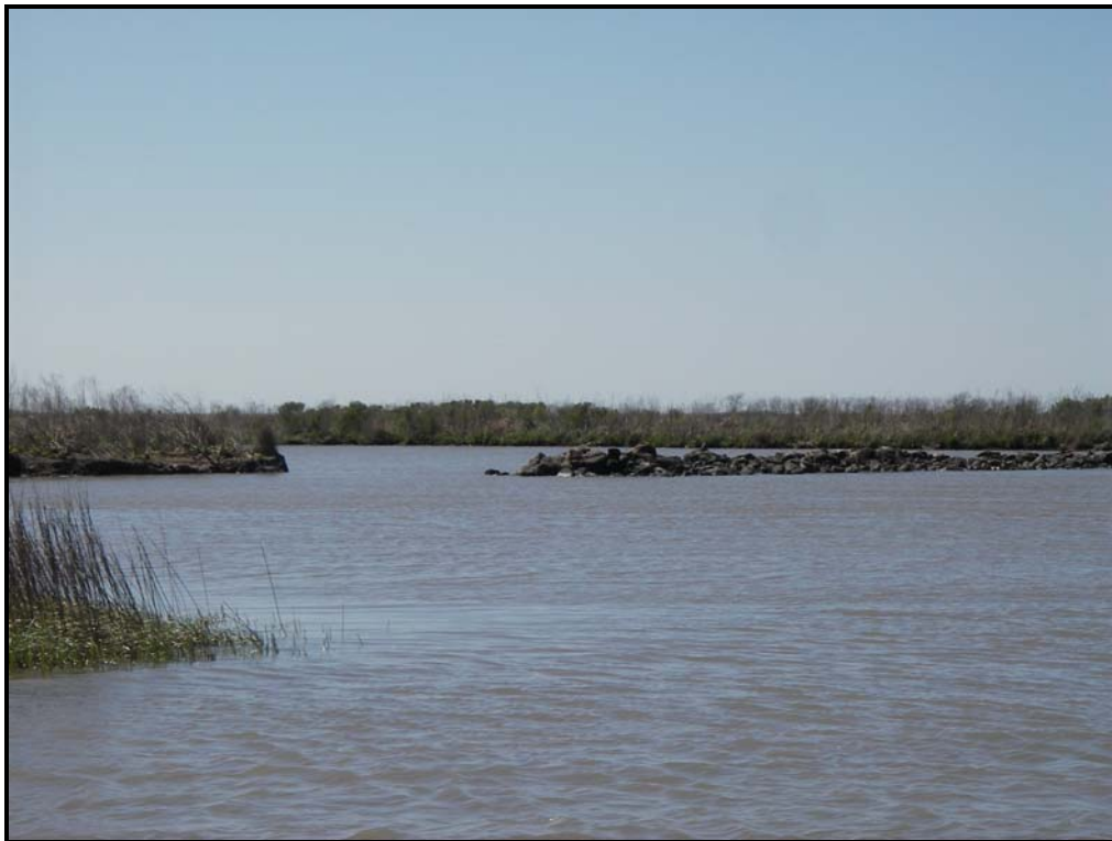
Photo 2, Closure No.2, View showing "flanking" cut on east end.
