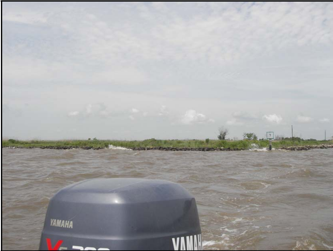
Photo 3 —south west side of Boston Canal at shoreline
