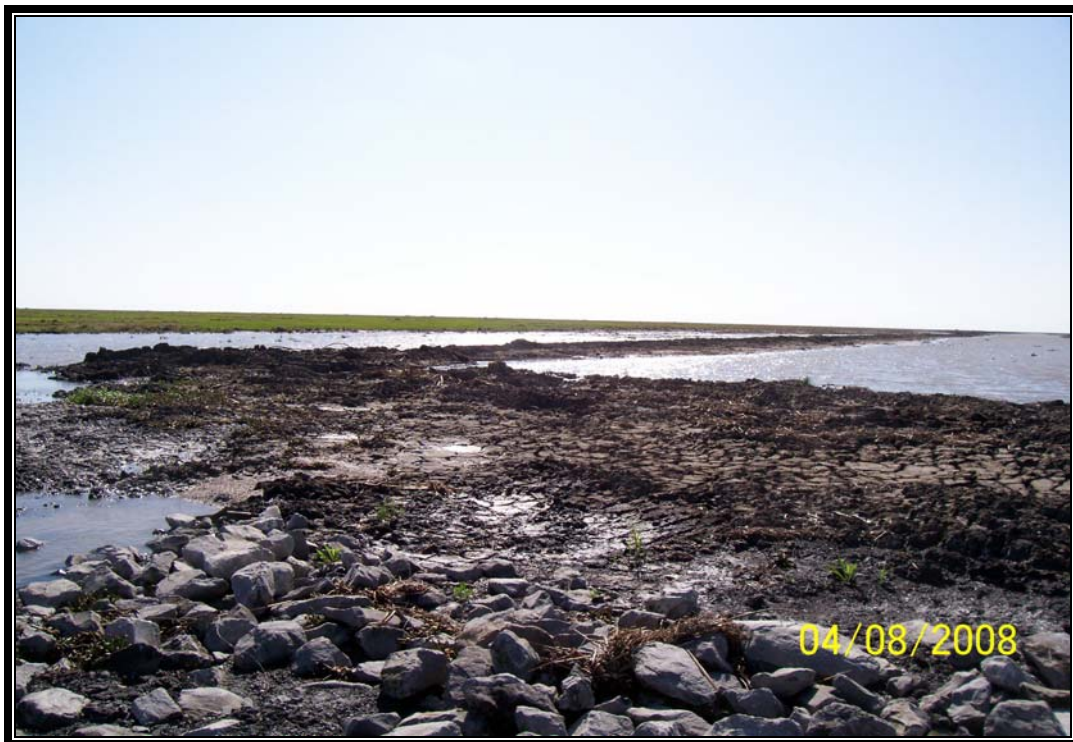
Photo No. 38 – view of containment levees along the old corridor to the Lake Chapeau disposal area. Containment was constructed during the Point au Fer Island Dedicated Dredge Project.
