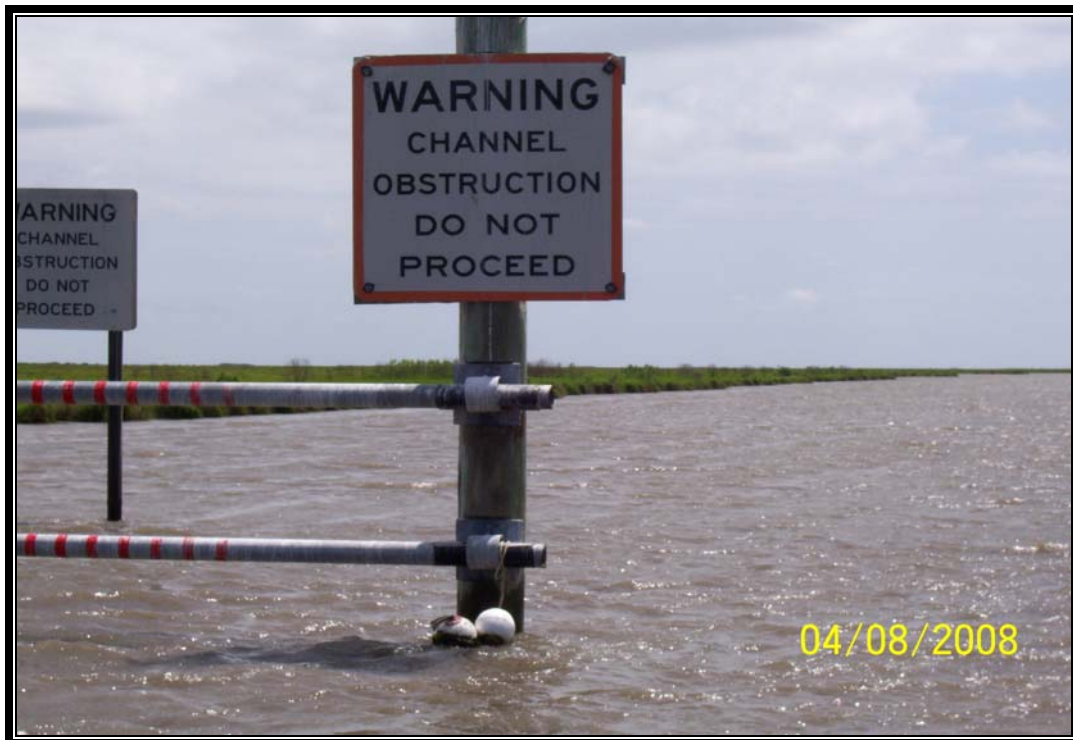
Photo No. 21 – view of the left center section of timber barricade system (Structure 6). The steel pipes were cut with torch.
