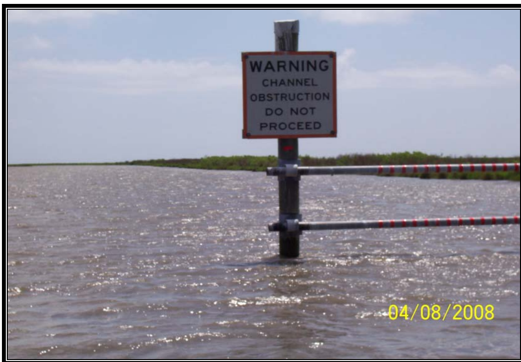
Photo No. 20 – view of the right center section of timber barricade system (Structure 6). The steel pipes were cut with torch.
