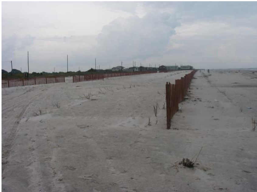
Figure 6b. View of the Sand Fencing and Vegetation Plantings at Station CS31-208 taken in October 2003. Note the double rows of fencing constructed here near the end of the project. The photograph is facing east.
