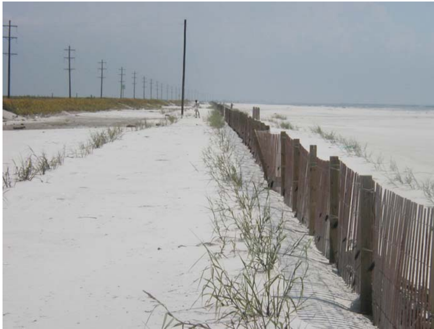
Figure 6a. View of the sand fencing and Vegetation Plantings at Station CS31-110 taken in October 2003. Note the dune formation already developing adjacent to the fences. The photograph is facing east.
