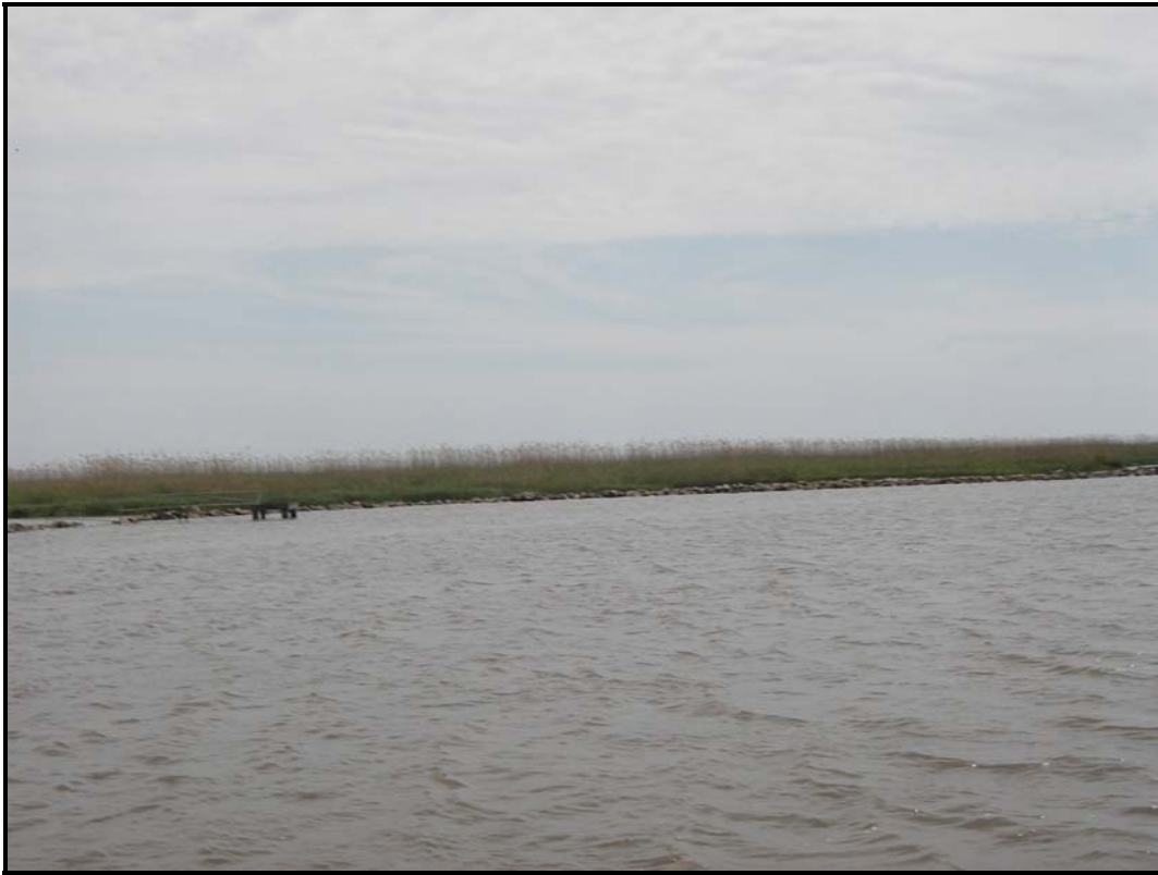
Photo 3 -typical rock dike section
