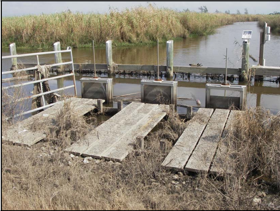
Photo No. 1, Structure No.1, inlet side.
