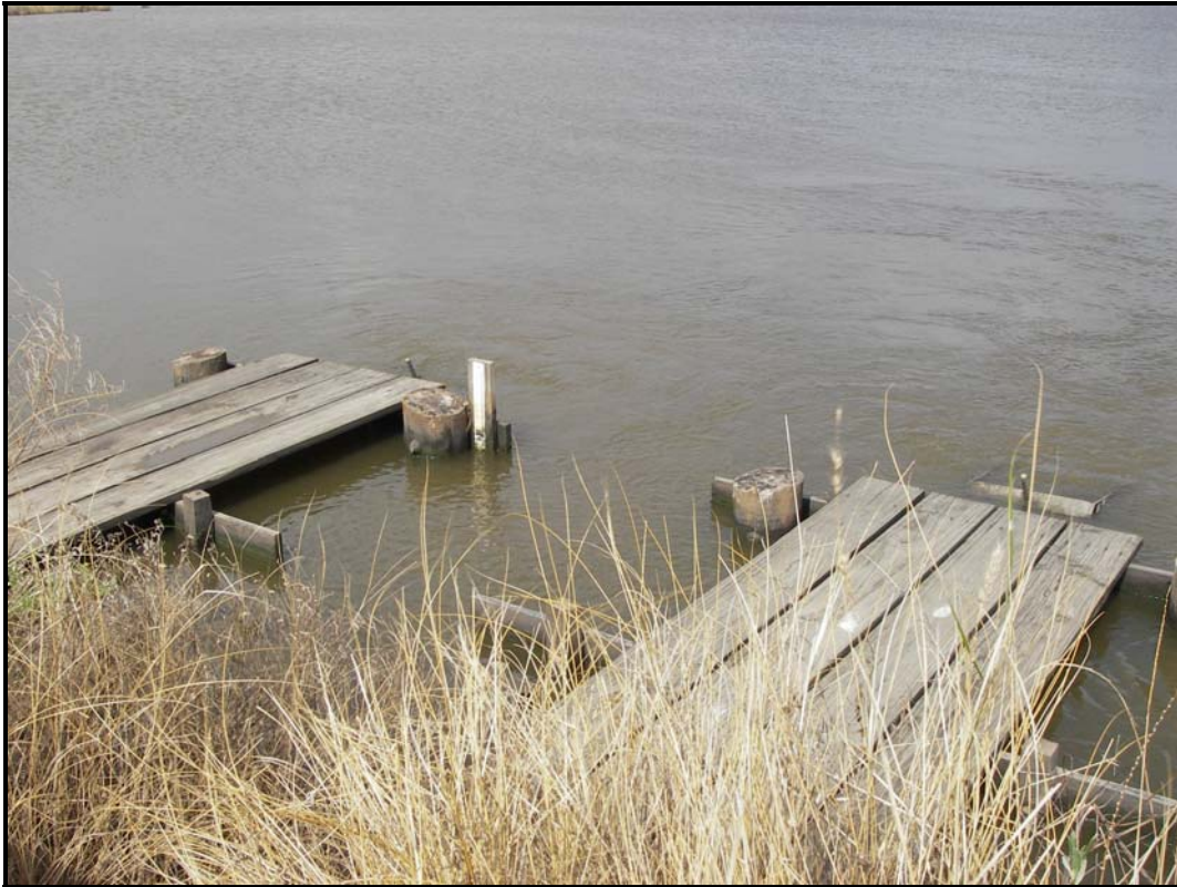
Photo No. 5, Structure No. 12, outlet side.
