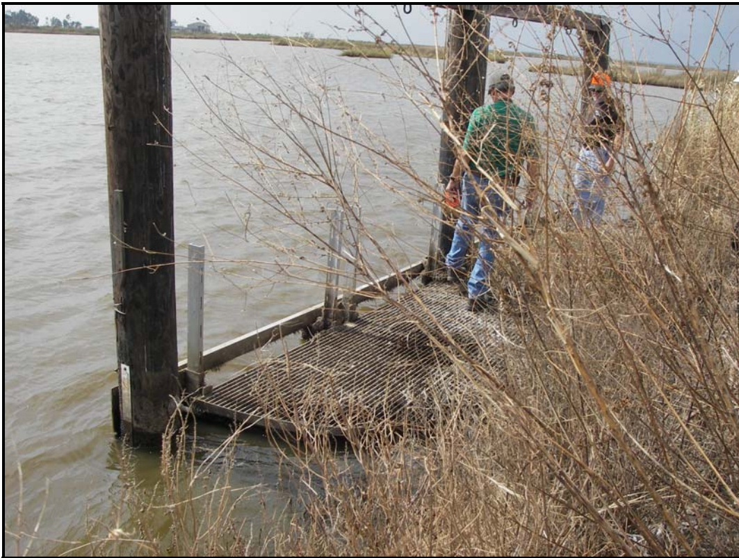
Photo No. 4, Structure No. 12, inlet side.
