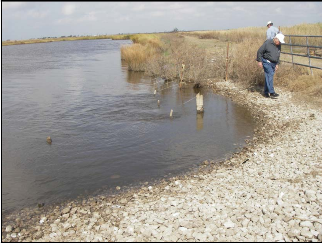
Photo No.3, Structure No.1, outlet side.
