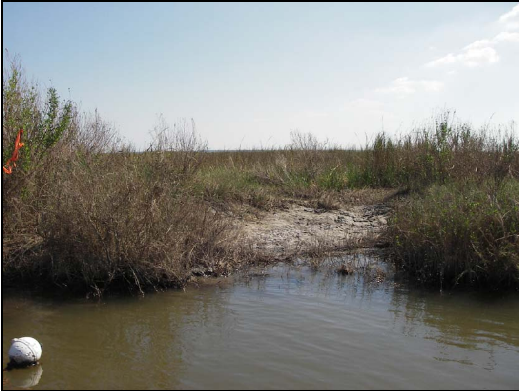
Photo No. 7, Typical levee erosion on eastern levee along Step Canal
