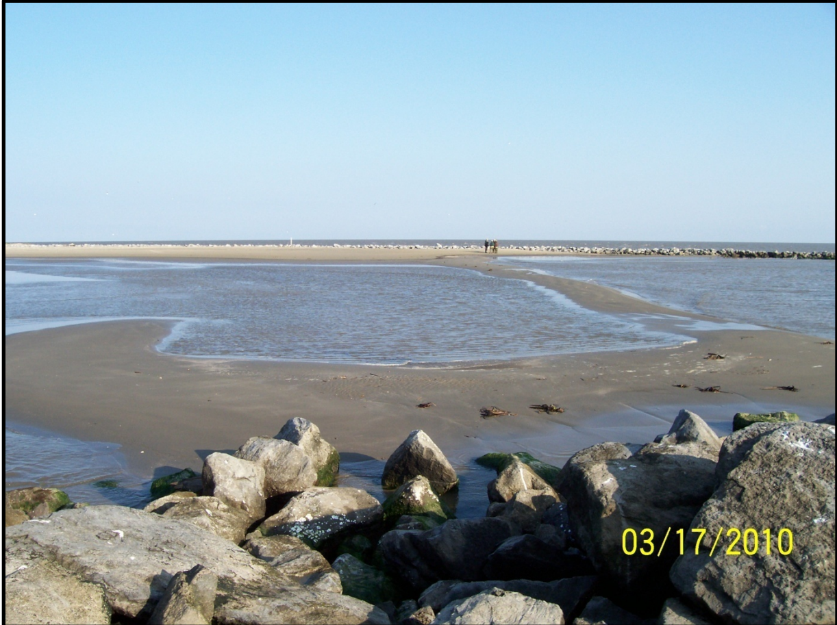
Figure 17. View of the tombolo forming behind breakwater 1 at the Raccoon Island Shoreline Protection/Marsh Creation (TE-48) project. Note the rock structure in the background is the groin.
