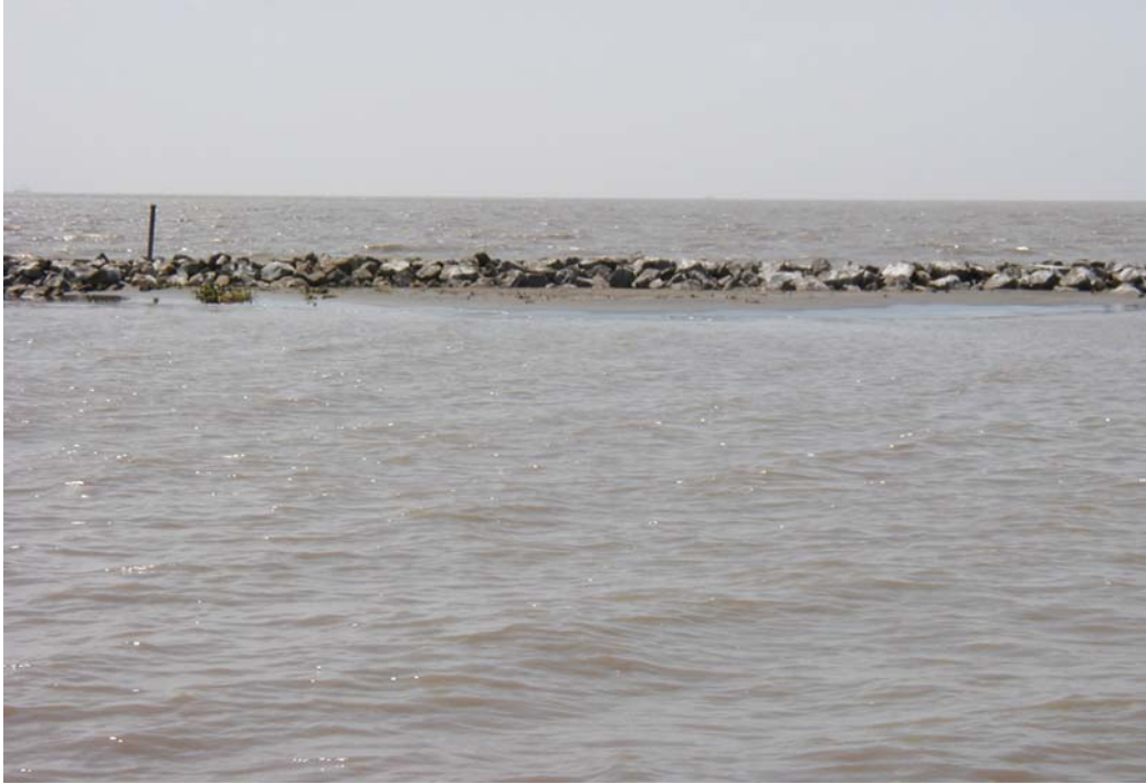
Figure 4. Segmented rock breakwater showing foreshore accreted sand approximately 6 mo. following construction.
