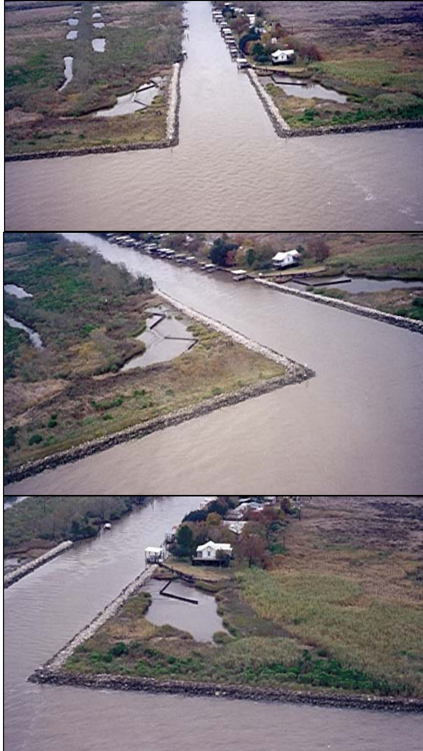
Figure 10. Boston Canal/Vermilion Bay Shoreline Stabilization (TV-09) rock breakwaters and sediment fences at the mouth of Boston Canal (January 2001).
