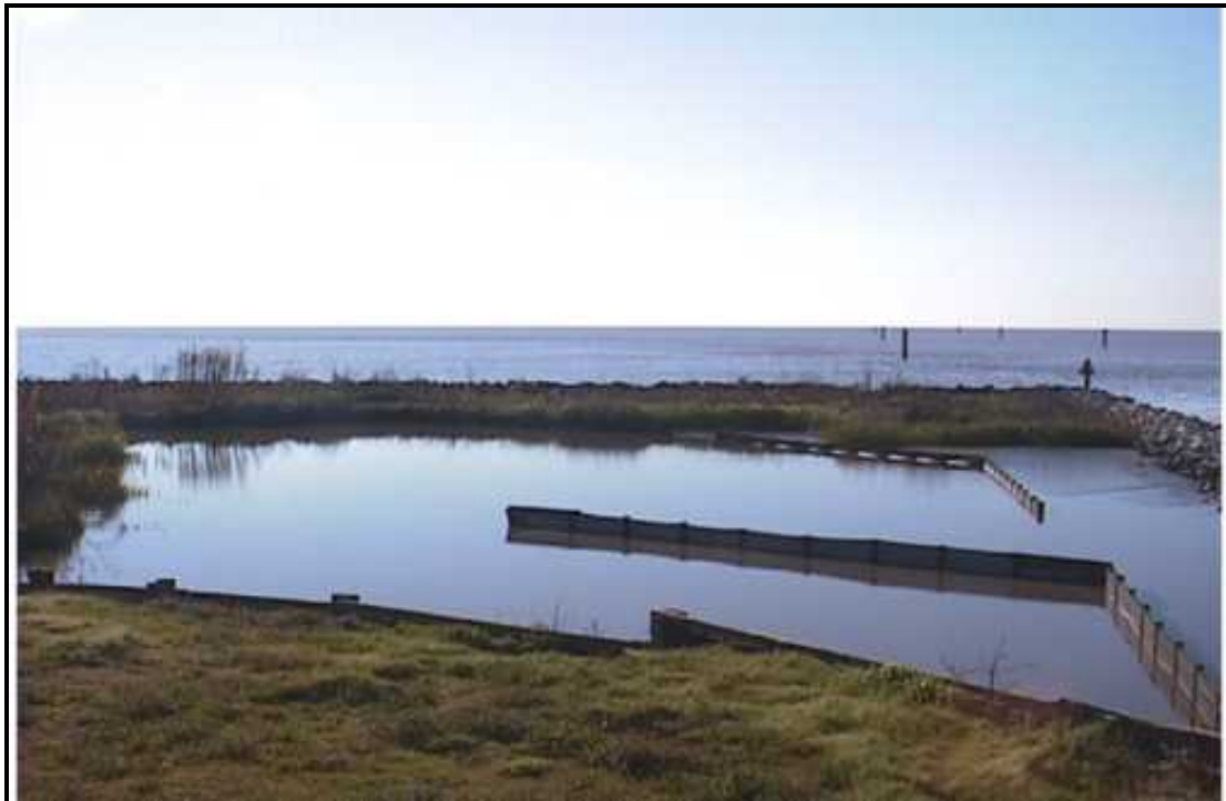
Figure 11. Boston Canal/Vermilion Bay Shoreline Stabilization (TV-09) photographs: (A) sedimentation behind the breakwaters December 1994: (B) vegetation growing behind the breakwaters in February 1998.
