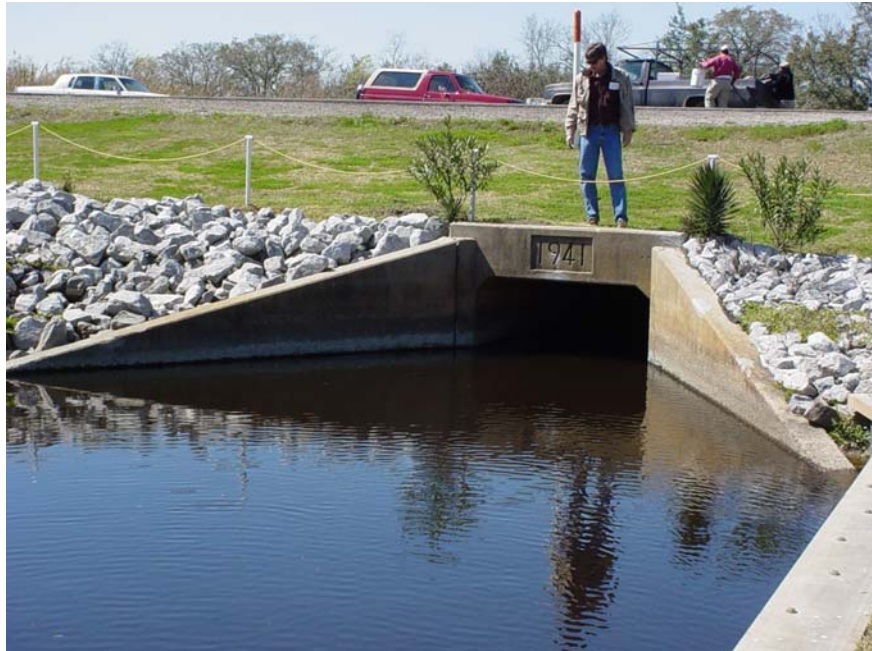
Photo No. 1 Pre-existing concrete box culvert under Hwy. 90 with adjacent stone riprap erosion protection placed in 2001.
