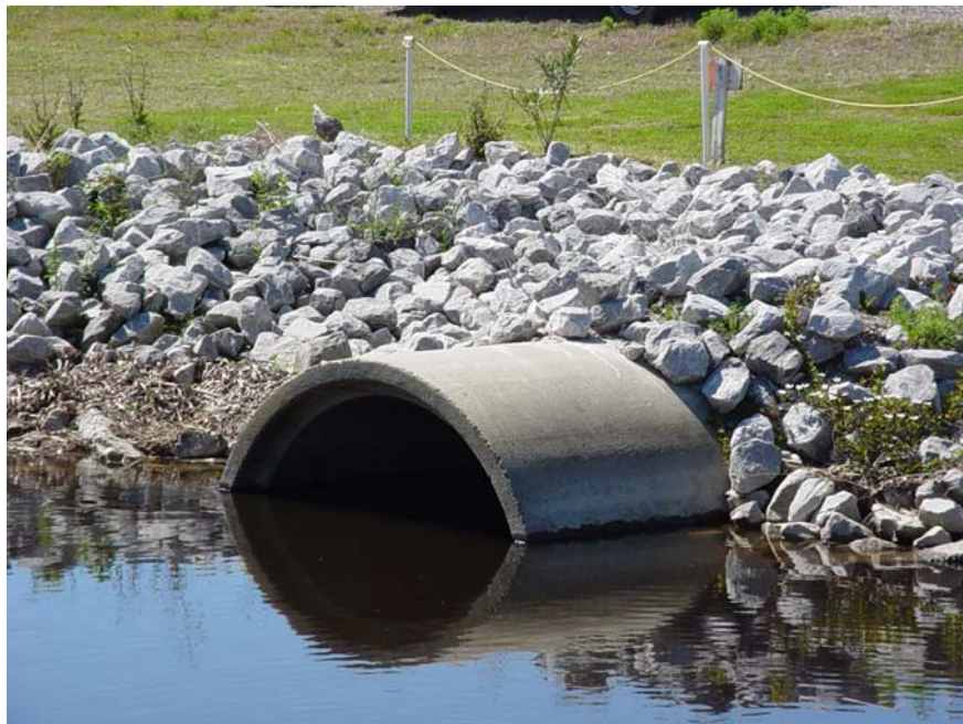
Photo No. 2 Round 72" concrete culvert under Hwy. 90 with stone erosion protection was completed in 2001.
