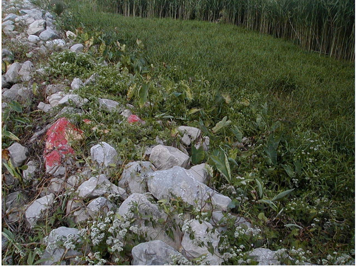
Figure 8. View of the Cameron Prairie rock dike showing naturalized vegetation colonizing the dike itself and the accreted marsh behind the dike. The red paint was used to mark the location of the shoreline marker for the DGPS survey.
