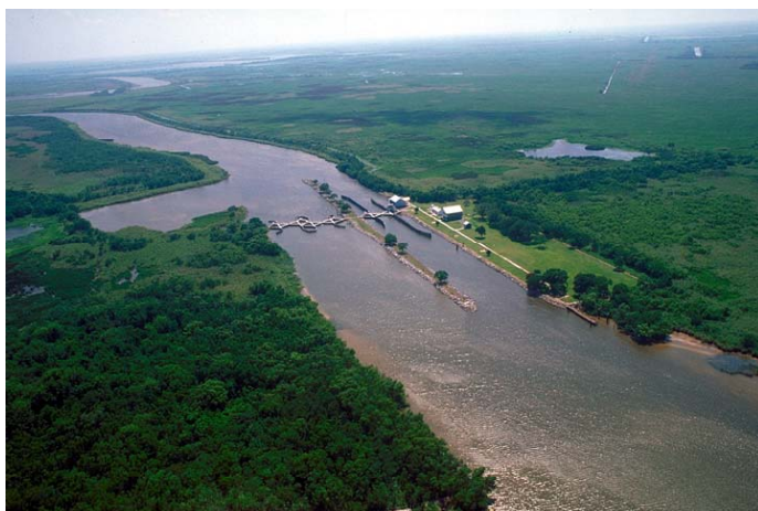
Figure 2. Catfish Point Control Structure, Mermentau River (USACE photo)
