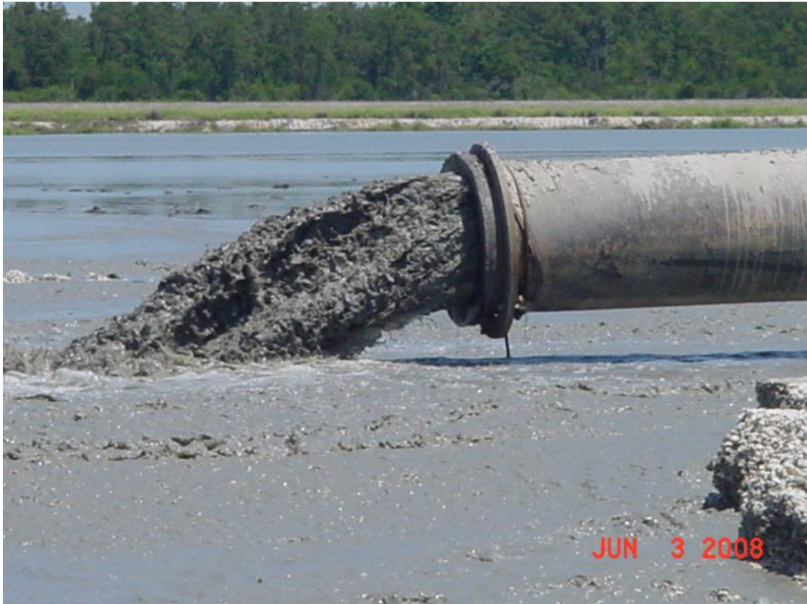
Placing dredged material
