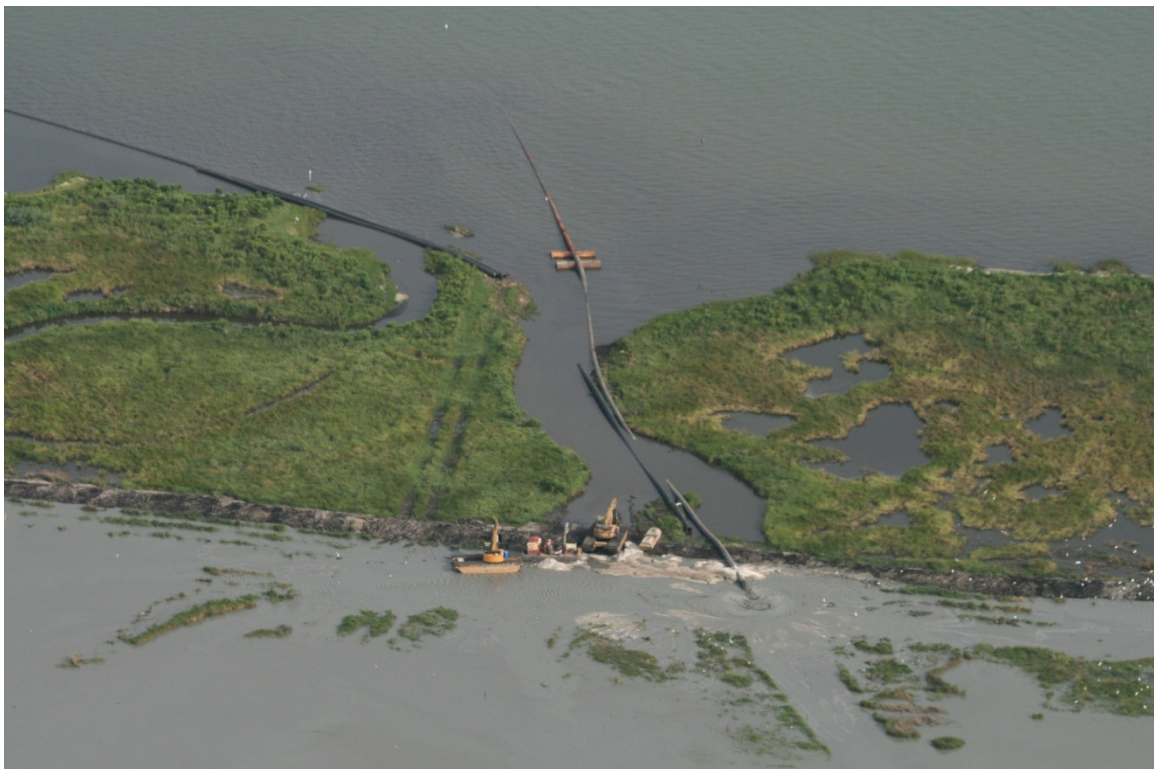
Placing dredged material
