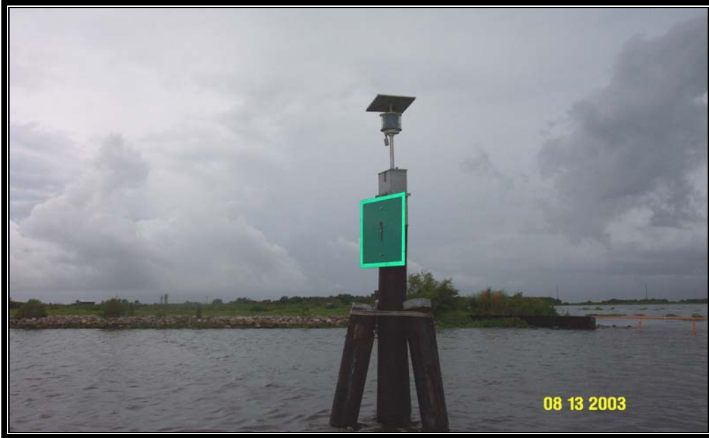
Photo of timber pile repair at Structure No.6 along Bayou Decade.
