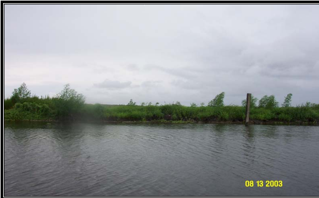
Breach 8 – Photo of levee repair along Superior Canal looking south.
