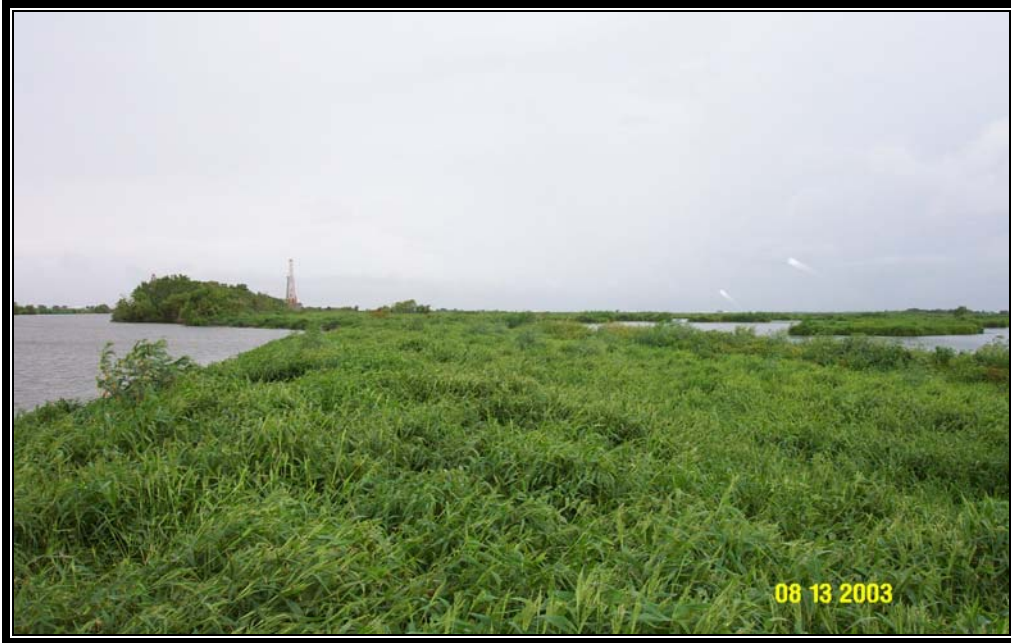
Breach 5 & 6 – Photo of breach repair along Turtle Bayou looking south.
