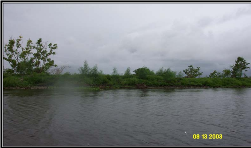
Breach 9 – Photo of breach repair along Superior Canal looking south.
