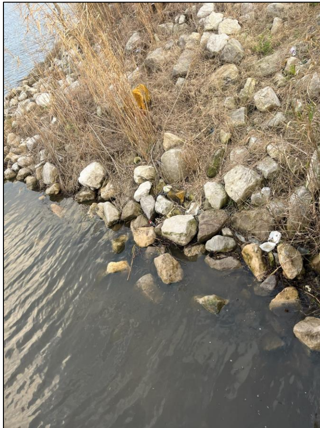
B8. East Side of Structure – South Riprap
