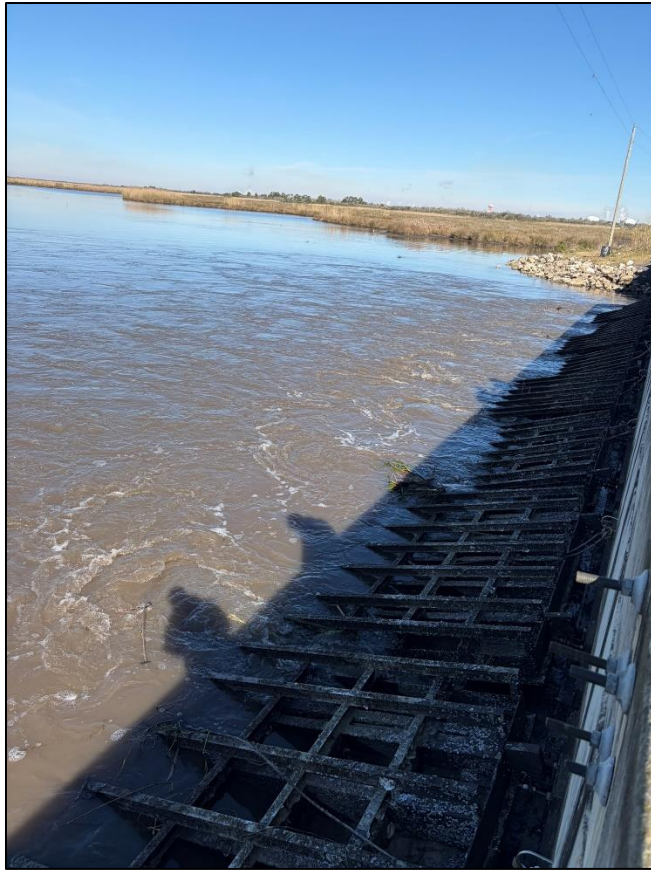
B1. West Side of Structure – Looking North
