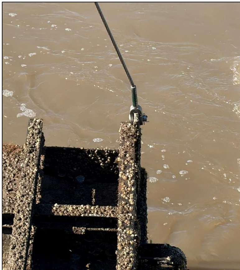
7d. Gate No. 7 – New Cable Installed
