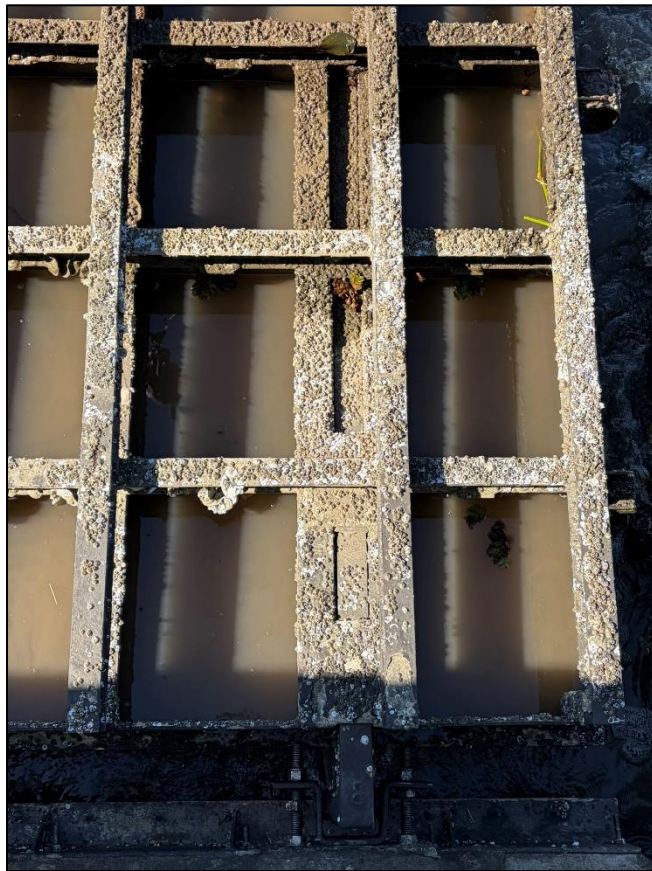
8g. Gate No. 8 – Hinge Assembly and Stop Plate – North Side
