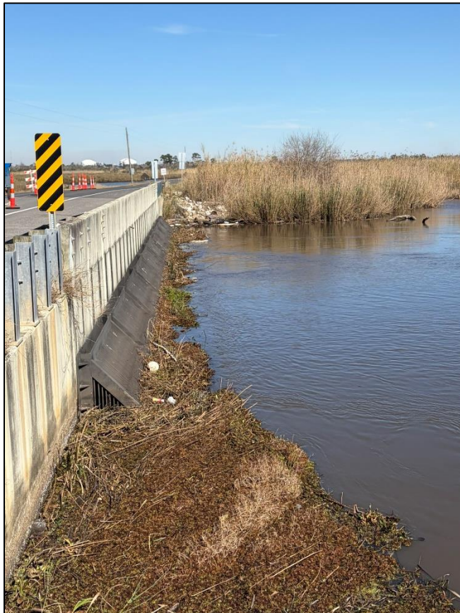
B6. East Side of Structure – Looking North
