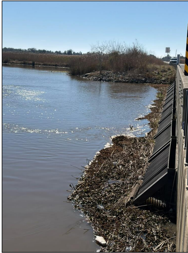
B7. East Side of Structure – Looking South
