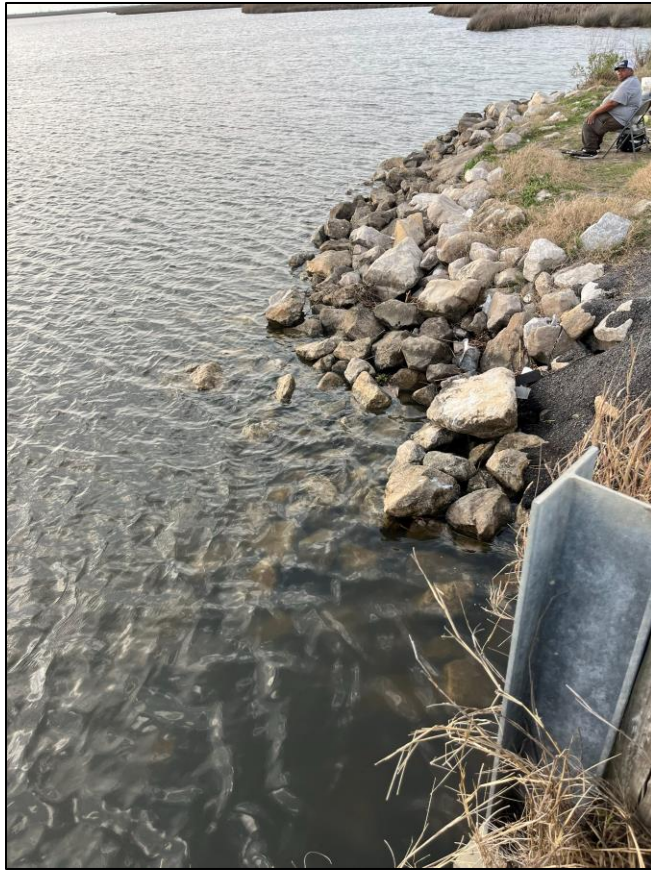
B3. West Side of Structure – North Riprap
