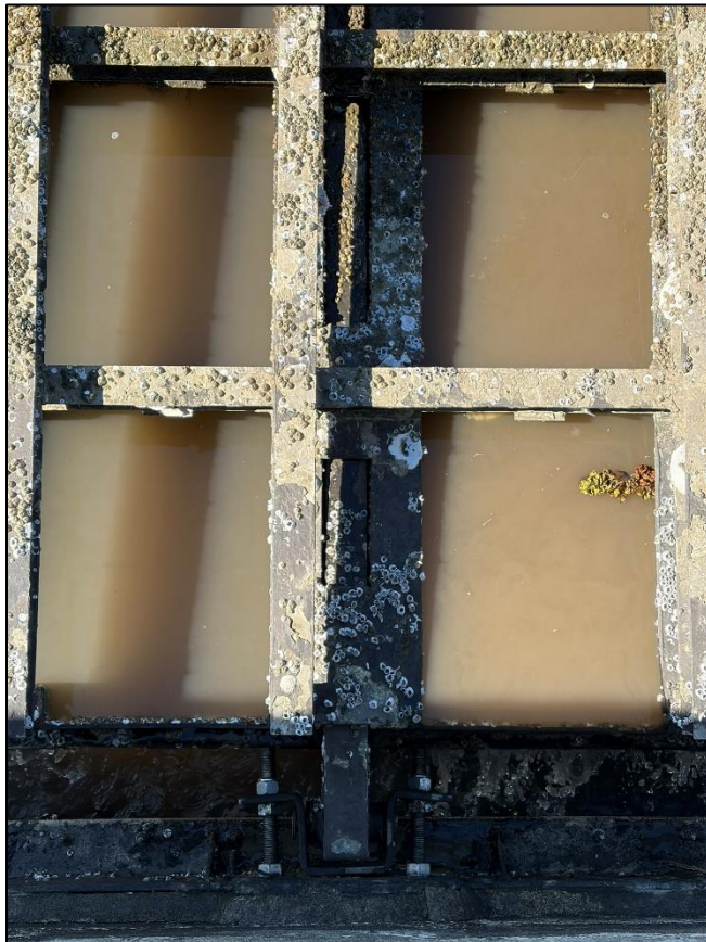
9f. Gate No. 9 – Hinge Assembly and Stop Plate – South Side
