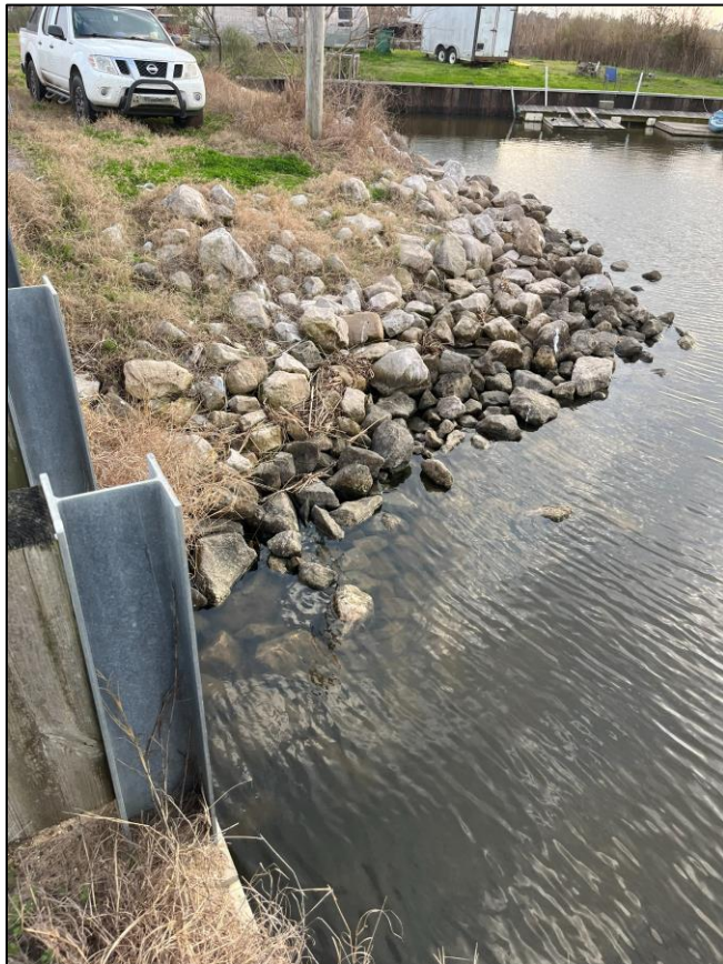
B4. West Side of Structure – South Riprap
