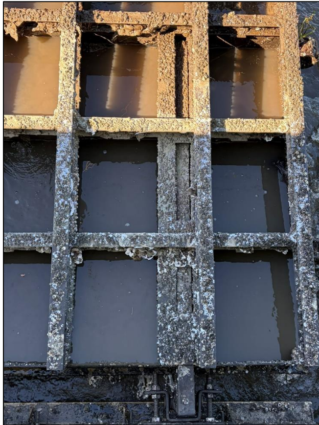
4g. Gate No. 4 – Hinge Assembly and Stop Plate – North Side
