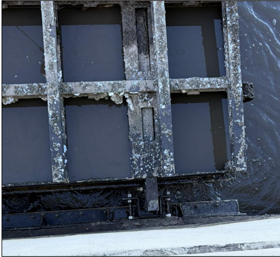
1g. Gate No. 1 – Hinge Assembly and Stop Plate – North Side
