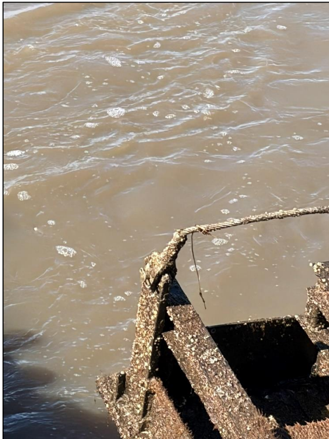
10f. Gate No. 10 –South Side of Gate - New Pin
