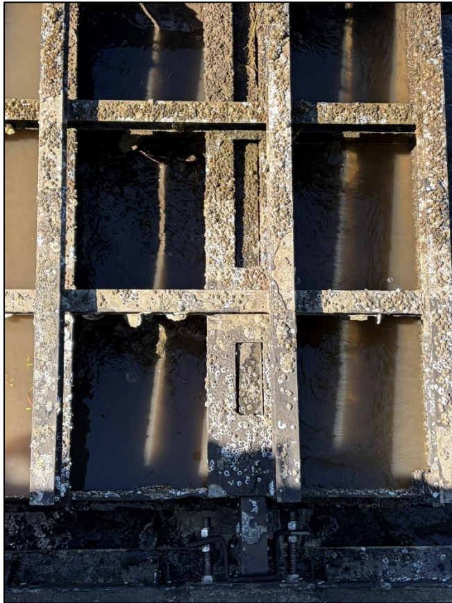
9g. Gate No. 9 – Hinge Assembly and Stop Plate – North Side
