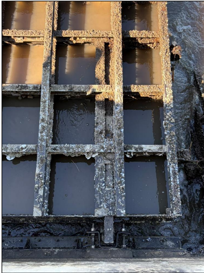
5g. Gate No. 5 – Hinge Assembly and Stop Plate – North Side
