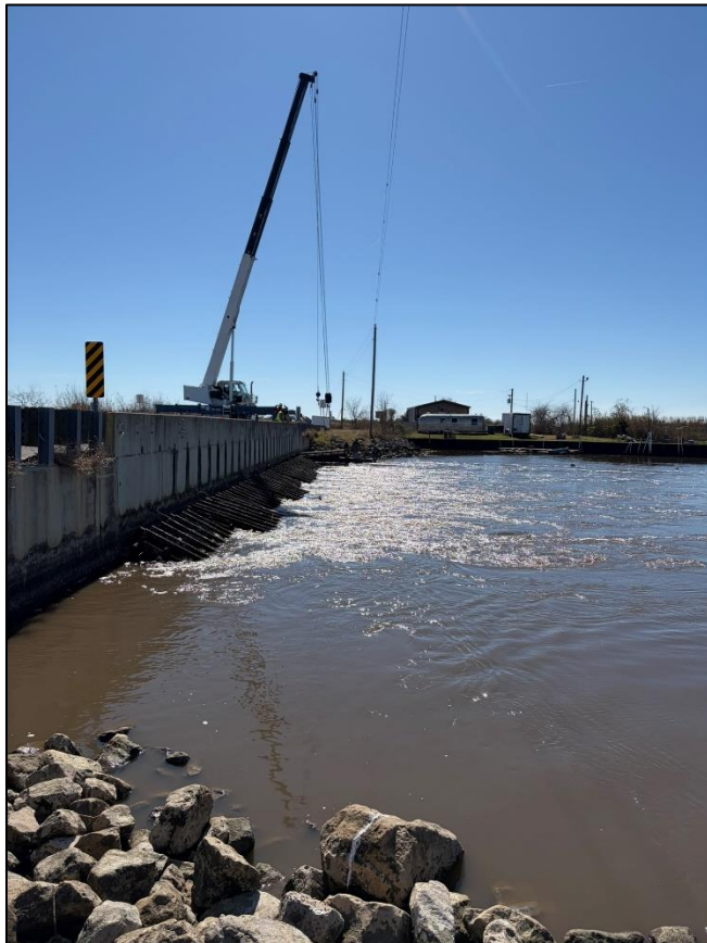
B2. West Side of Structure – Looking South
