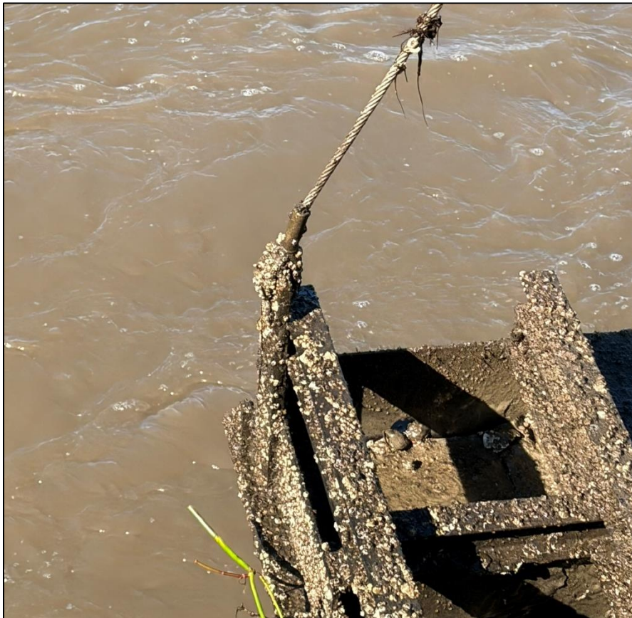
3f. Gate No. 3 – Lifting eye, shackle and cable - South side of Gate
