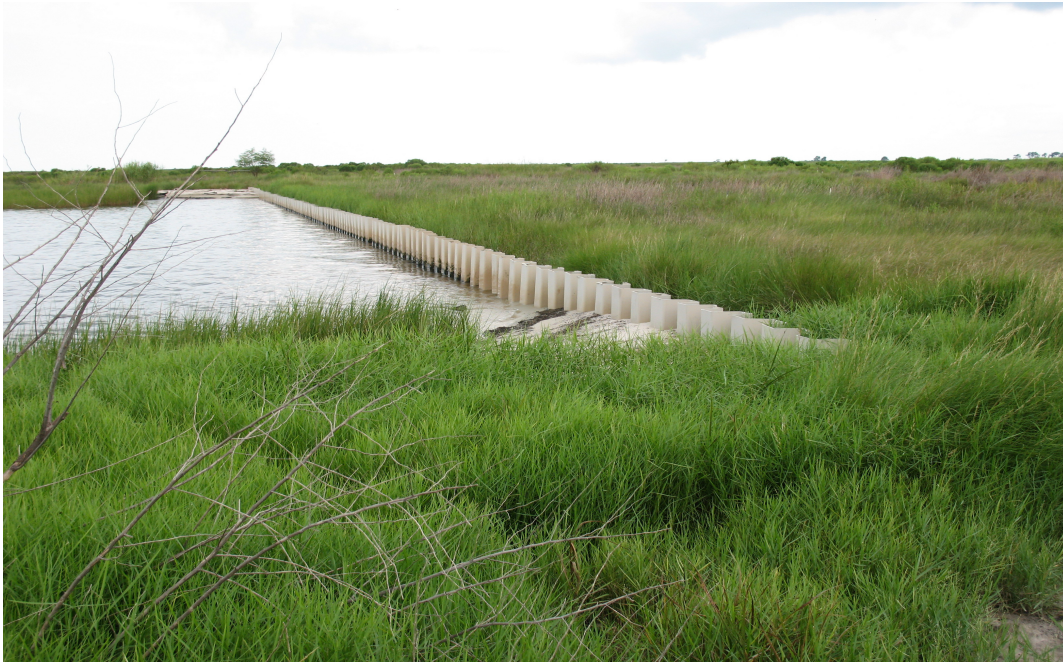
Area “D” --One of three reaches along lake rim where vinyl sheet pile was placed to prevent lake from encroaching into marsh creation area.
