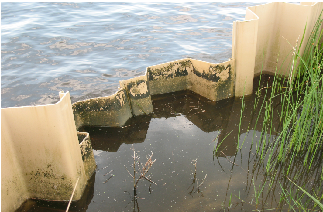
Area “D” --Hunters cut notch in vinyl sheet pile for easy boat access from the lake into the new marsh creation areas.
