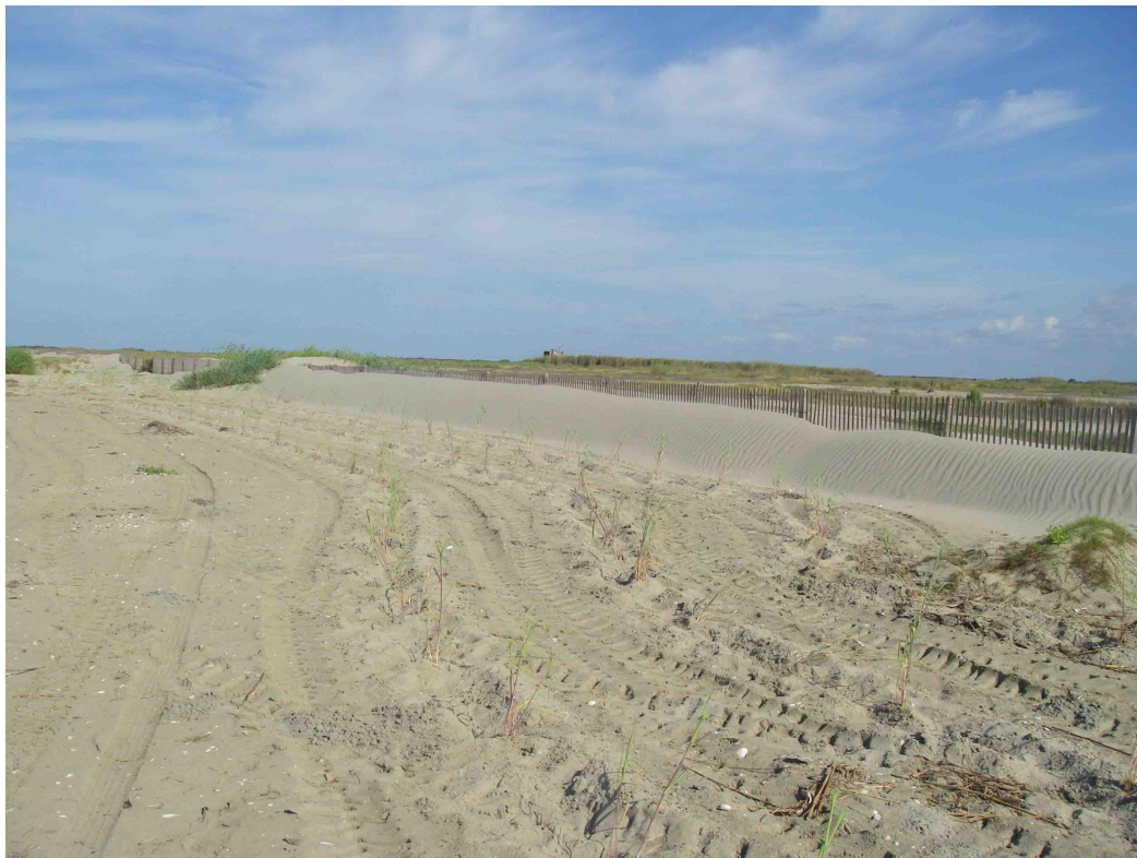
Photo #2 – Old Fencing (BIMP January 2010), note sand deposition.
