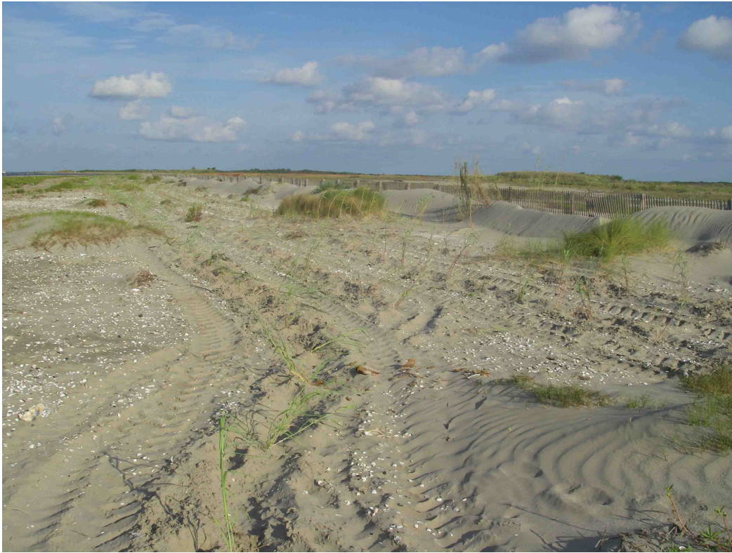
Photo #1 – Old Fencing (BIMP January 2010), note sand deposition.
