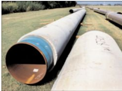
Figure 1: Concrete Pipeline Coasting
