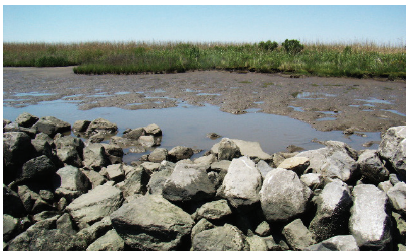
Figure 4. The shoreline protection provided by the rock dike in the ME-13 project area has been effective in reducing shoreline erosion and has increased overall land acreage since construction.
