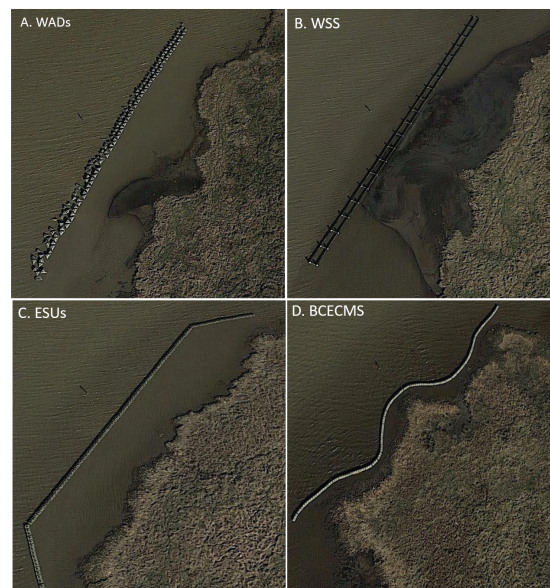
Figure 24. A close up image of each section of structures shows a better view of mudflat formation behind the WADs and WSS.
