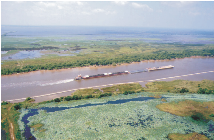
Figure 2. An aerial image of the CS-22 project along the GIWW
