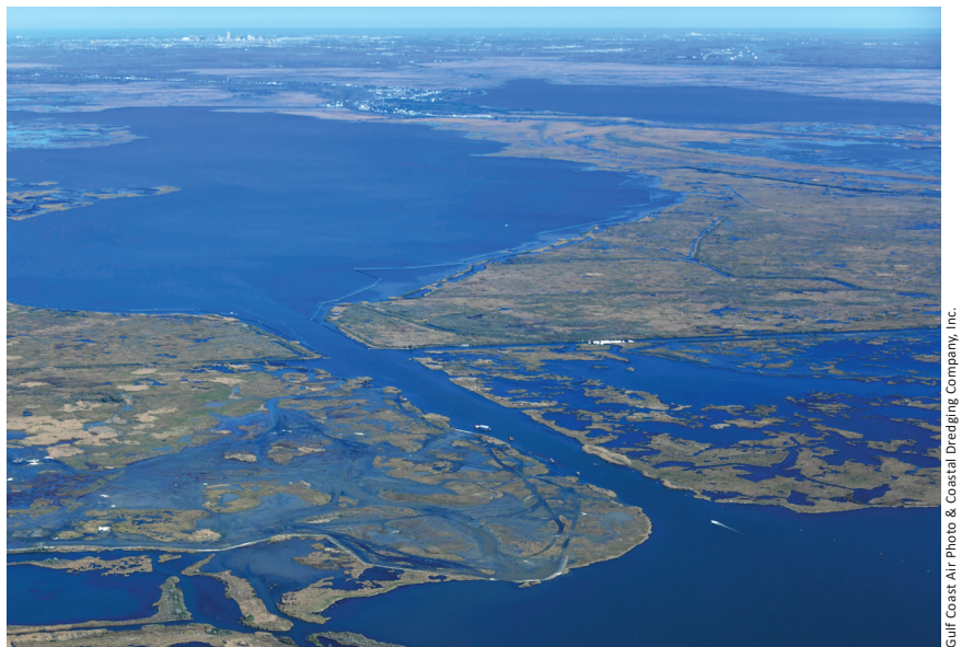
CWPPRA projects provide protection to coastal communities. The Northwest Turtle Bay Marsh Creation (BA-125) project consists of approximately 700 acres of marsh created with dredged material from Turtle Bay or Little Lake. Roughly six to seven miles to the northeast are the towns of Lafitte and Jean Lafitte, fishing communities rich in culture and located in the middle of the Barataria estuary.
