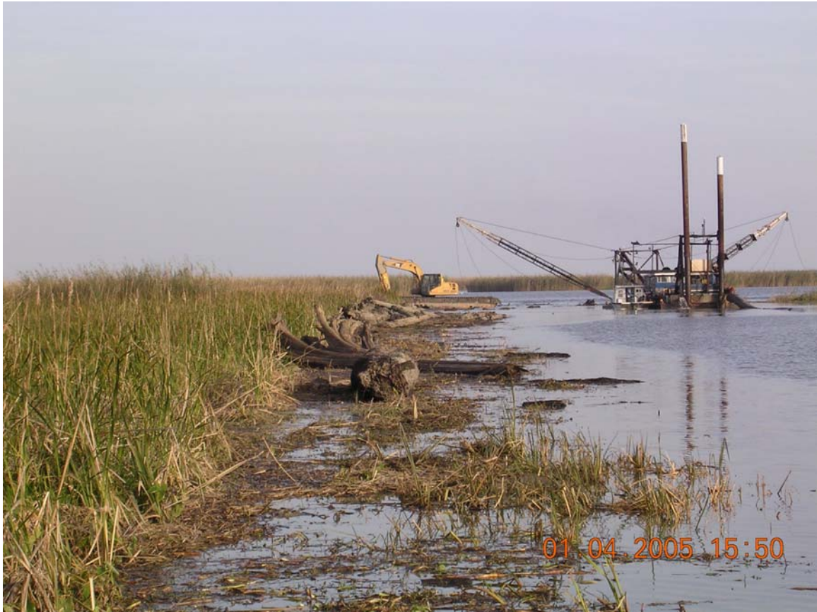
Photo 15. Logs and debris removed from Crevasse 11.
