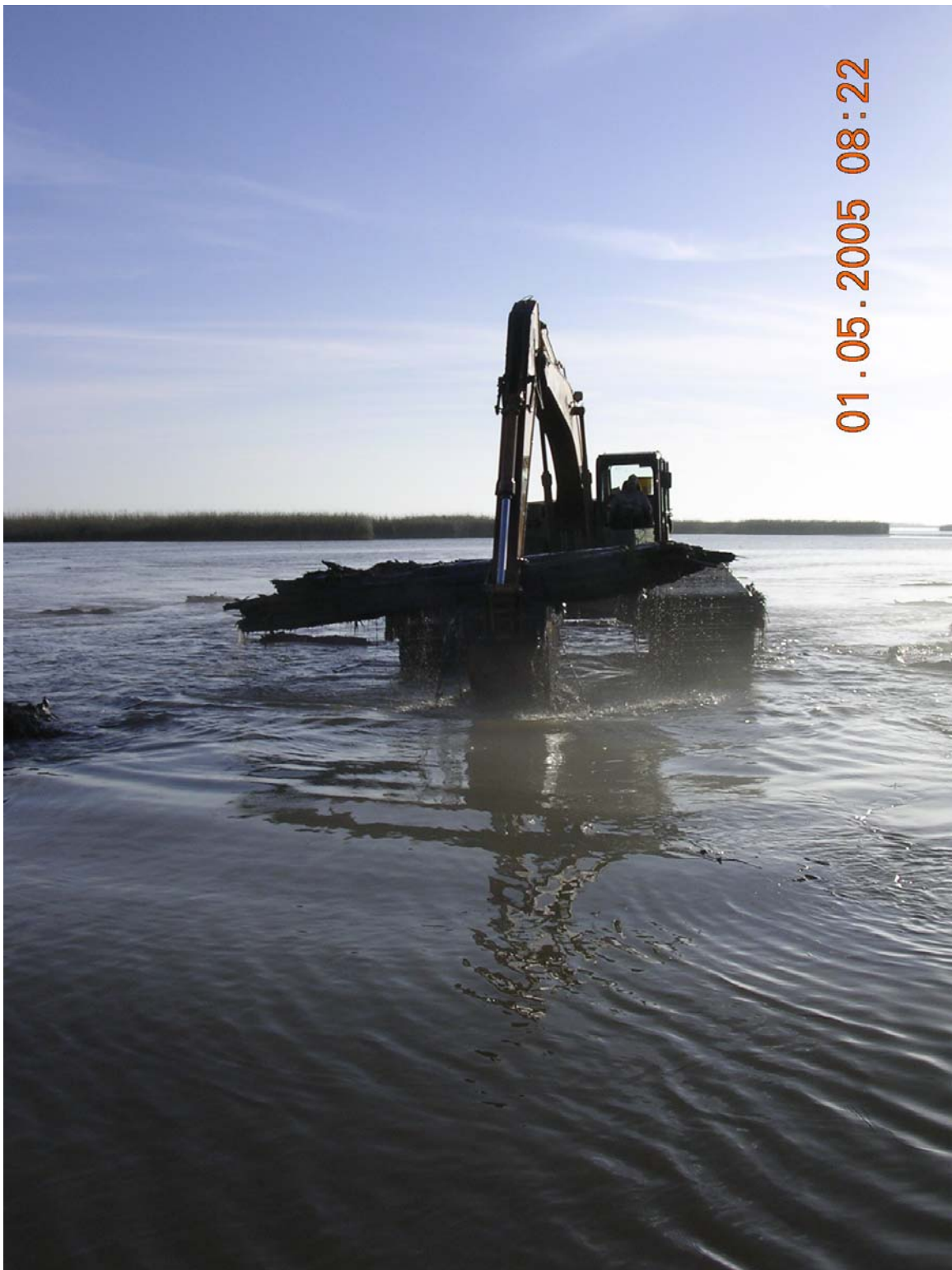
Photo 16. Marsh excavator removing submerged logs ahead of dredge.
