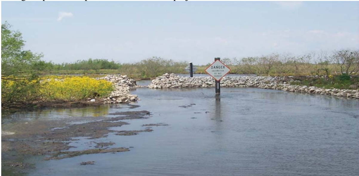
Picture1. Site #32 looking west, showing the breach in the rock closure caused by vandals, possibly trappers, in the area.
